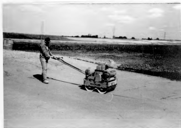
Figure 14. Compacting a Liner Lift (Indiana)
