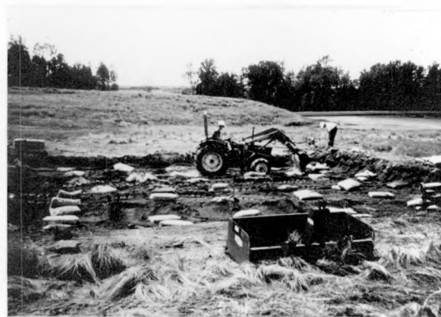
Figure 9. Adding Cement and Lime (Texas)
