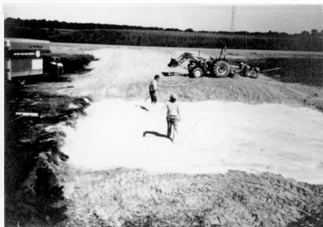
Figure 12. Spreading Cement and Lime (Indiana)
