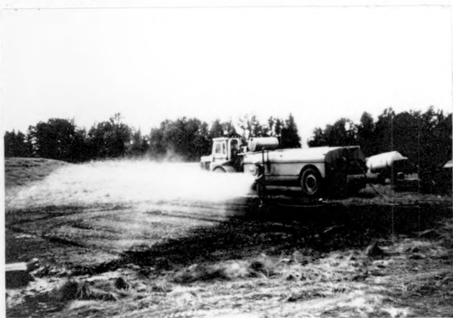
Figure 10. Adding Water to Liner Mix (Texas)
