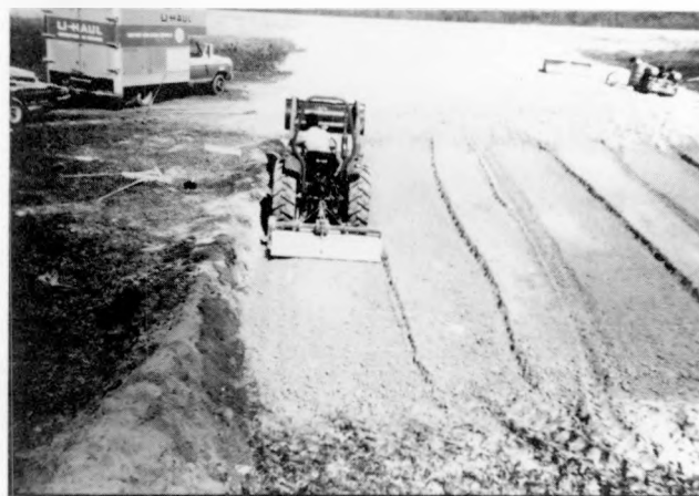
Figure 13. Tilling In Additives (Indiana)
