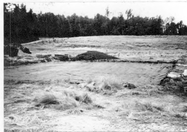
Figure 11. Completed Liner Lift (Texas)
