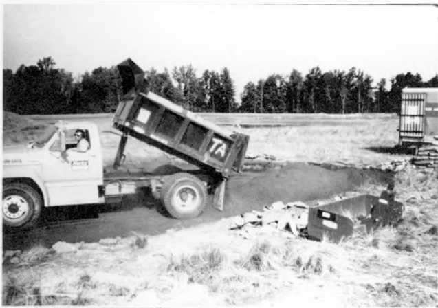
Figure 8. Spreading Fly Ash (Texas)
