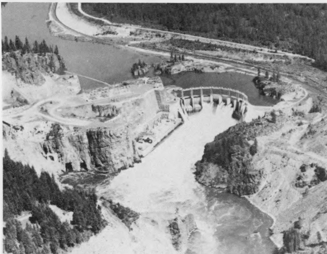
Figure 9. Cabinet Gorge project has an outdoor type powerplant.
