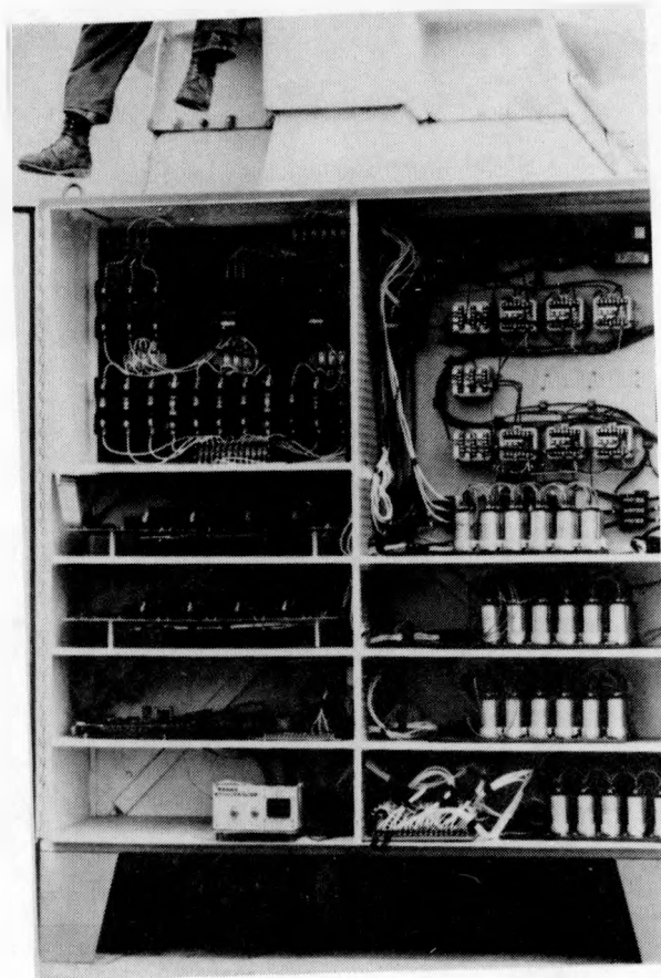
Figure 3.2: Closeup View of 50-kVAR. OL-APFC
