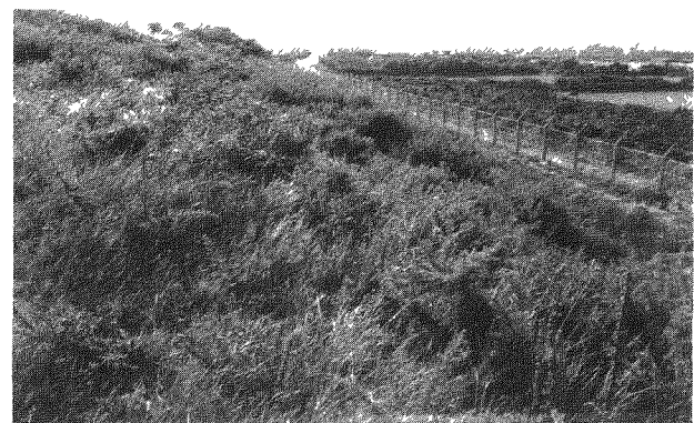
d. A completed Earth Mounded Concrete Bunker at the Centre de la Manche, France. Upon completion of backfilling operations, the entire mound is covered with a thick layer of impermeable clay, which in turn is covered by a layer of topsoil. The surface of the mound is stabilized by planting native vegetation which not only stabilizes the soil but encourages drying.
