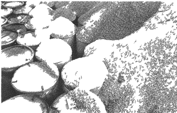
c. Cohesionless backfill material is placed periodically during construction to fill the voids between drums, thus reducing the potential for future settlement, and increasing the stability of the mound.
