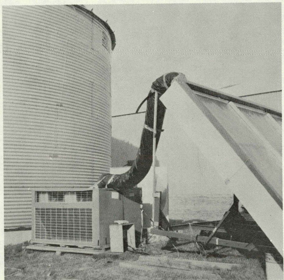
Figure 2. Flexible duct used to duct heated air from solar collector to drying fan and 17.58 kW heat pump used in the experiment.
