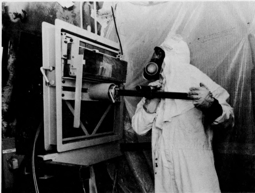
FIGURE 3.23. Semi-Remote Abrasive Wheel Cutting at Top of Seventh TSP
