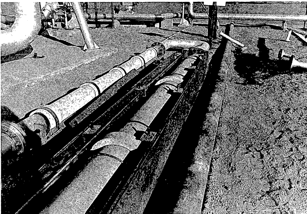
Figure 18. Polymer impregnated concrete and asbestos cement pipe installed at East Mesa but not as yet connected to brine system.
