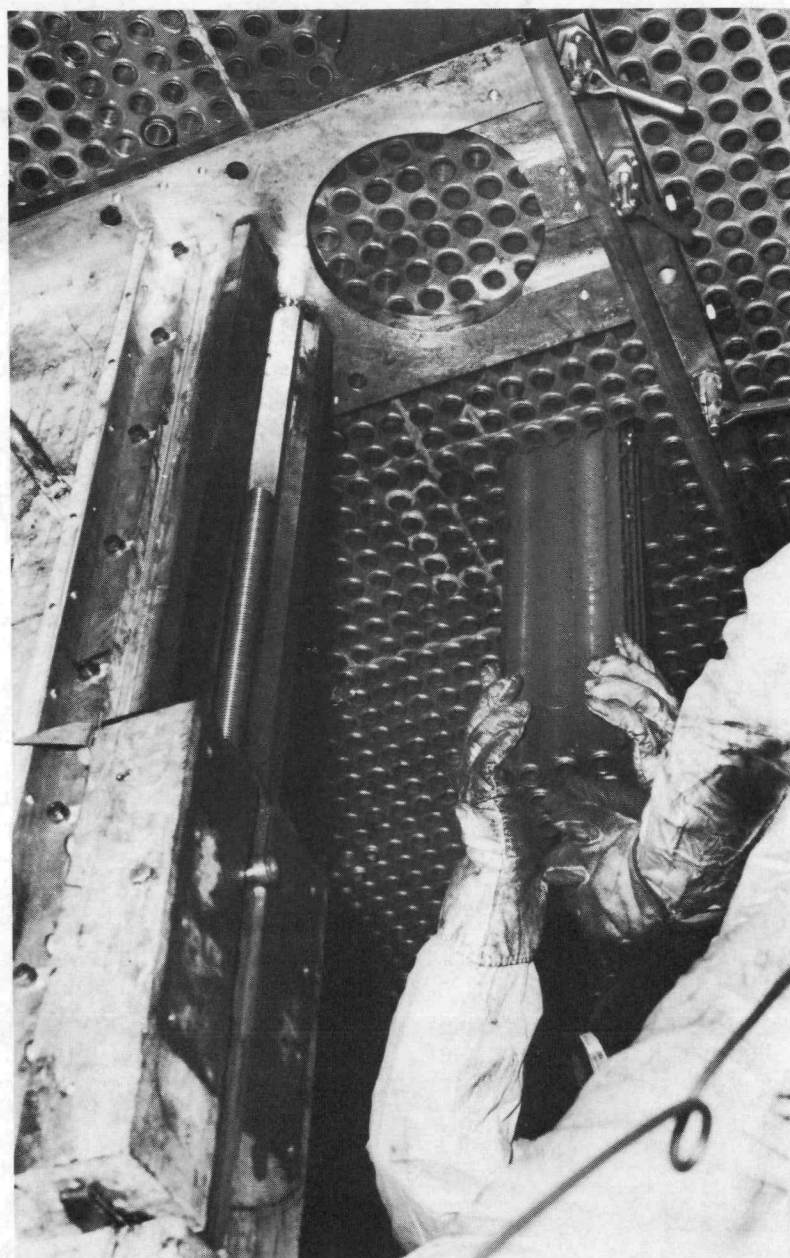
FIGURE 2.14. Removal of Hot Leg Tube Sheet Section
