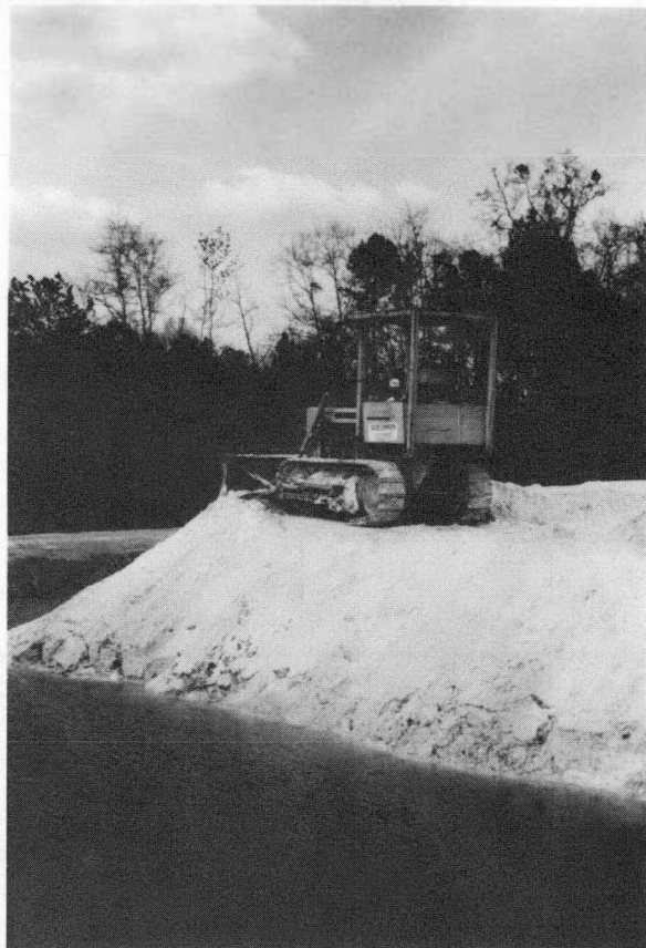
Figure 8-7 Leveling Top of the Stack 3/27/79
