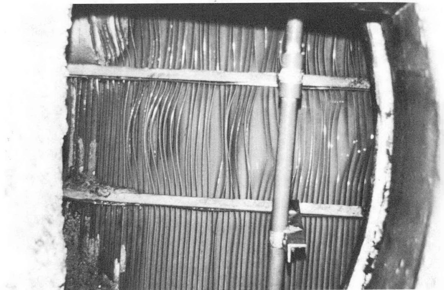
Figure 5-35 Before and After Washing Mist Eliminators (Three Days Since Previous Wash) (Damaged Sections Due to CT-101 Program)
