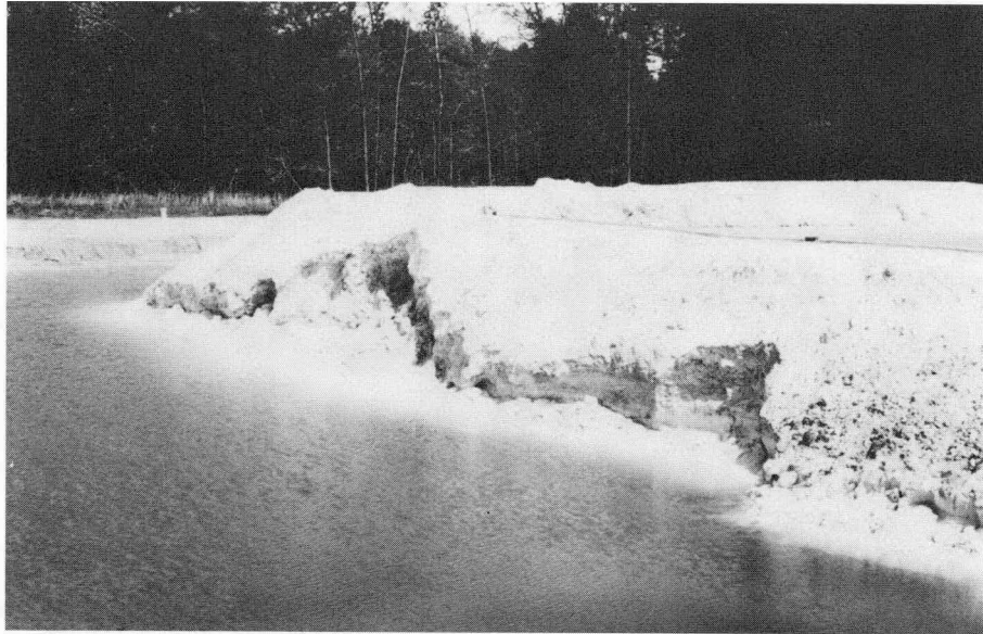
Figure 8-10 East Wall Sloughing At Water Line 4/27/79
