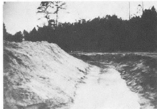
Figure 3-11. Raising North Wall of Cast Gypsum Dike
