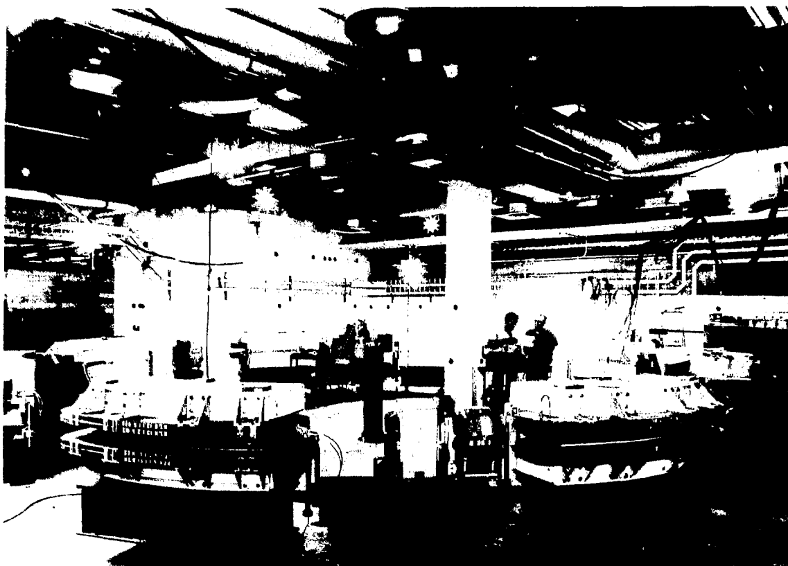
Figure 2. The Booster Synchrotron in process of assembly.
