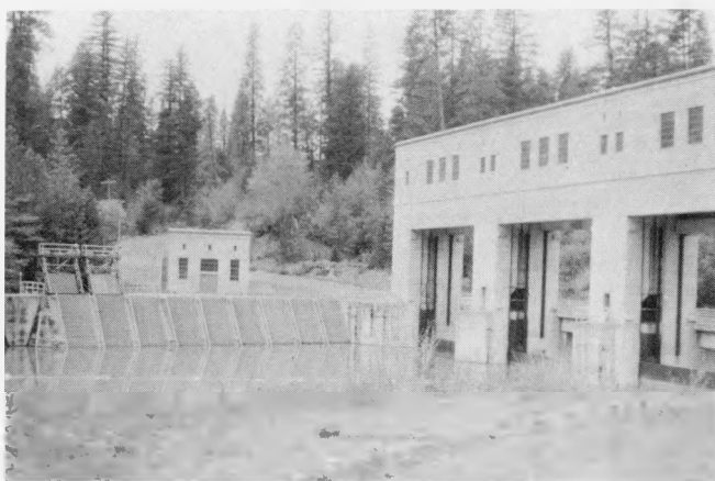
Figure 32. Upstream view of Pit No. 5 diversion dam shows intake structure at left and spillway gate structure with control house at right.
