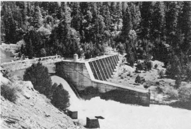
Figure 30. Pit No. 4 diversion dam and spillway.
