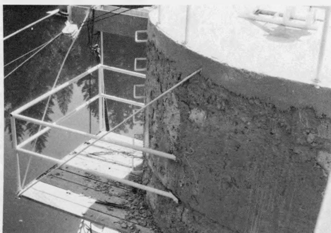
Figure 35. Spalling at Pit No. 4 diversion dam.
