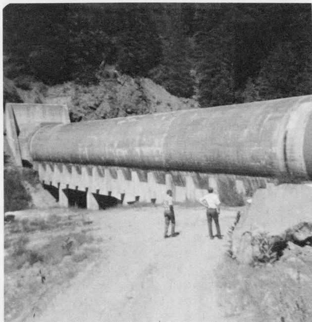
Figure 27. Concrete pipe over Rock Creek.
