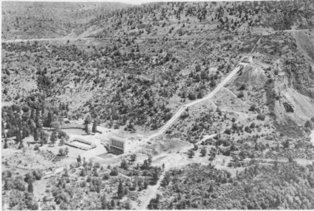
Figure 12. Pit No. 1 powerhouse and penstocks leading up to power tunnel outlet.
