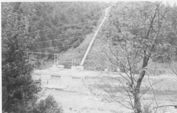
Figure 17. James B. Black outdoor-type powerhouse and penstock.
