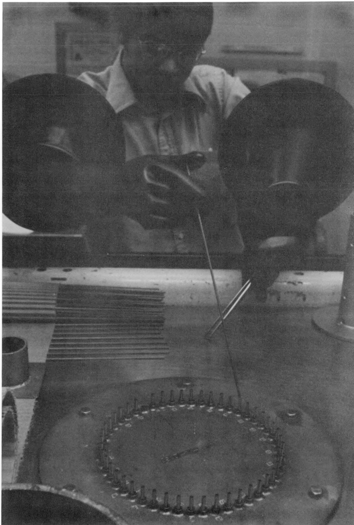
Fig. 22. Loading Fuel Slug into Jacket
