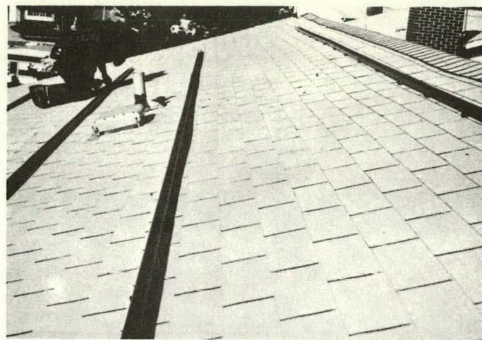
Figure 3-8. Attach UNISTRUT to Roof
