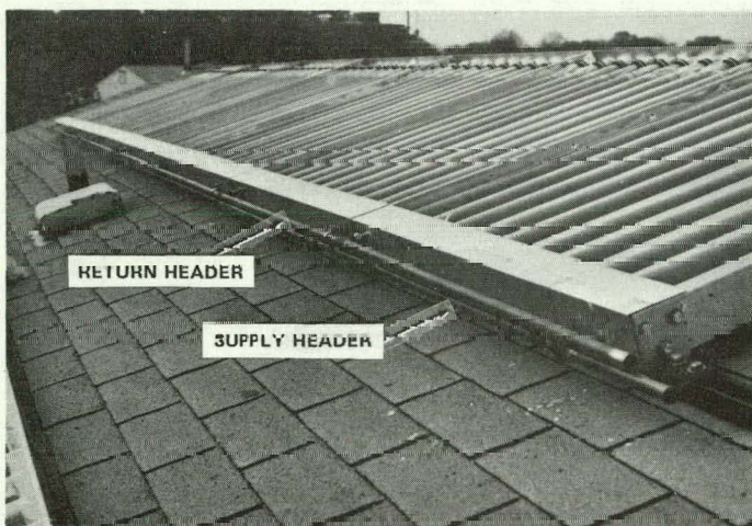
Figure 4-4. Install Headers
