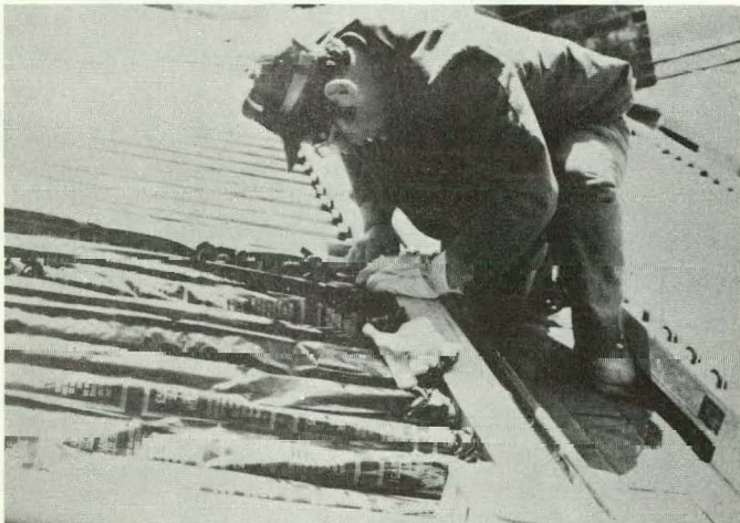
Figure 5-2. Firmly Seat Grommet into the Collector
