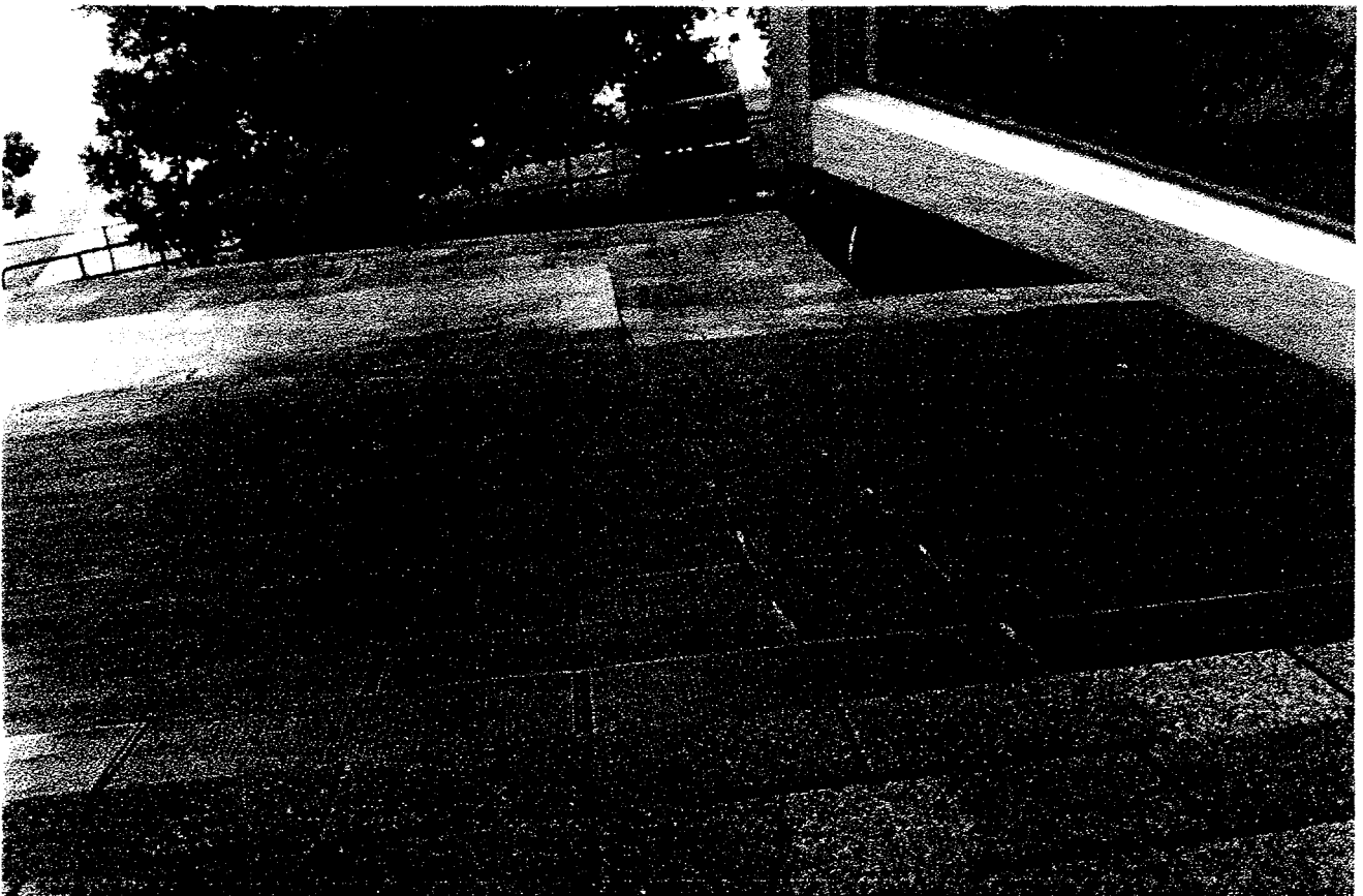
Fig. 1.C.3-4. Array after final installation. The ends of the modules fit together giving an almost indiscernible seam.
