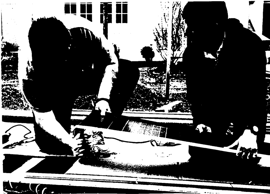
Fig. 2.C.1. Before installation the module is trimmed to the precise length and the end folded over to wrap around the sheathing at the eve of the roof.
