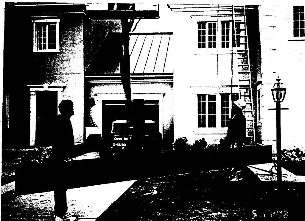
Fig. 2.C.2. Two workmen easily holding the lightweight flexible PV metal roofing module prior to loading the module onto the lift to be carried up to the roof.
