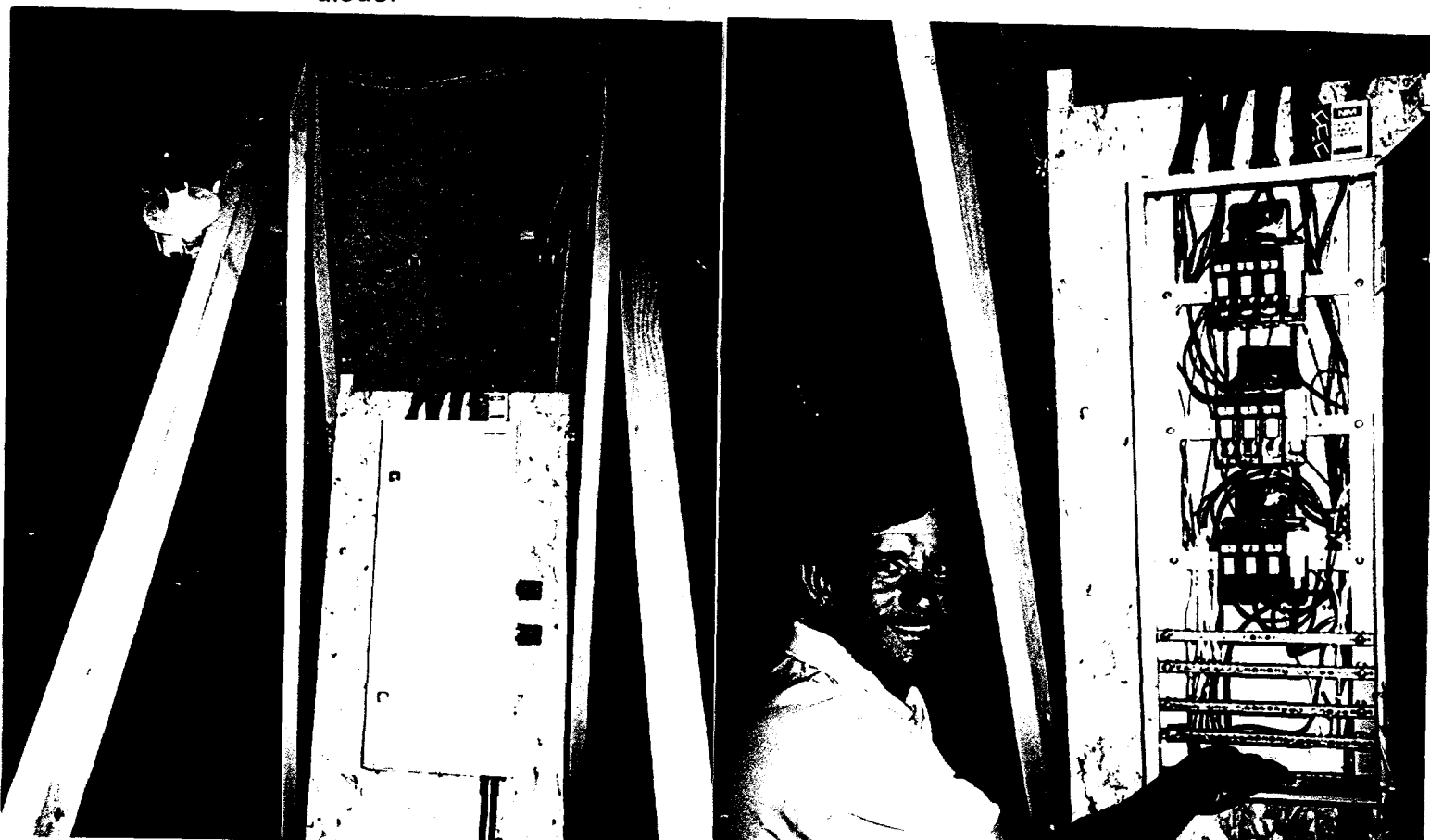
Fig. 2.B.4-5 Photograph of the Combiner Box in the NAHB 21st Century Townhouse. The nine inputs from the J-boxes are at the top of the box; the three output strings to the charge controller leave from the bottom of the box.
