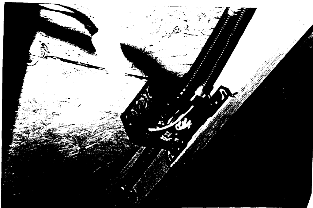
Fig. 2.B.3. Photograph of one of the 9 Junction Boxes in the NAHB Townhouse in which two modules are series connected. Two conduits, one from each module, can be seen entering the box at the top; one conduit leaves the box and goes to the combiner box. The J-Box also has a series blocking diode.
