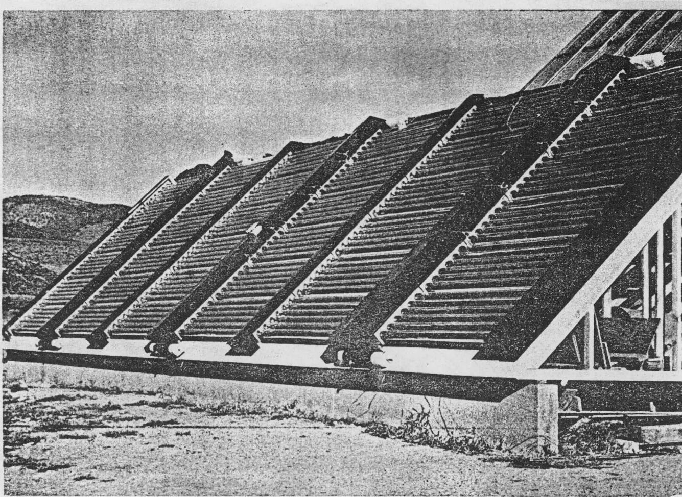
Figure 2.2.1. Corning Evacuated Tube Collectors
