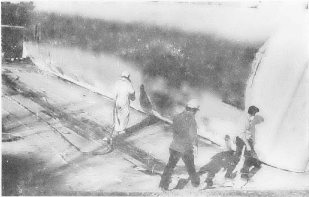
Fig. 3-15 Spray Application of Insulation to Tank
