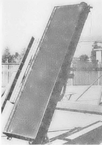
Fig. 3-4 Collector Assembly
