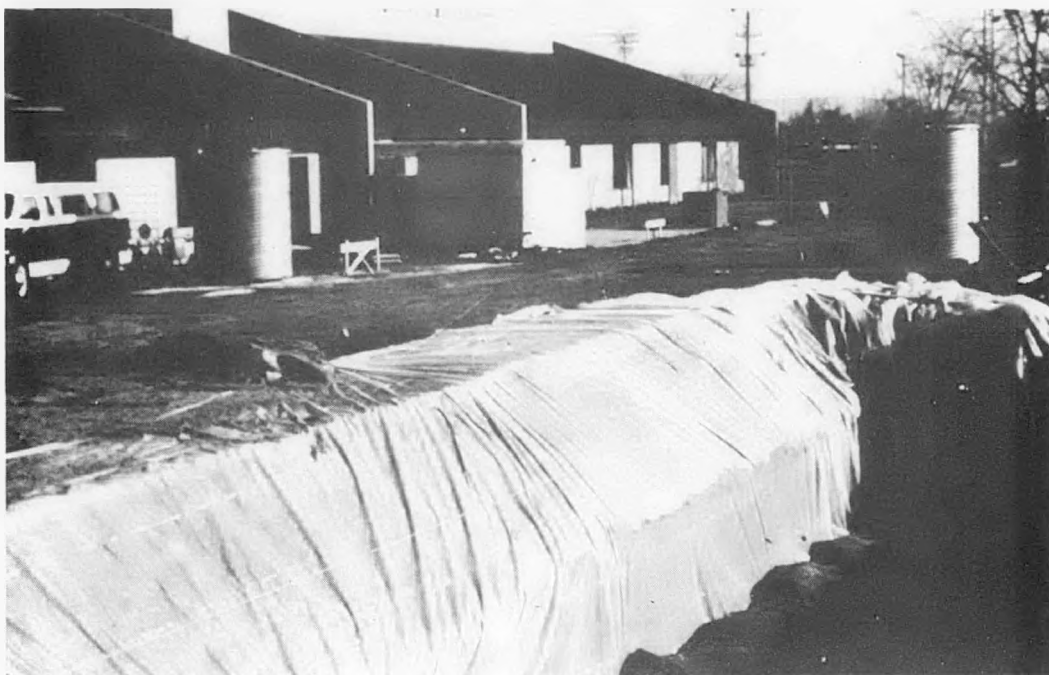
Fig. 3-21 Ground Preparation for Tank
