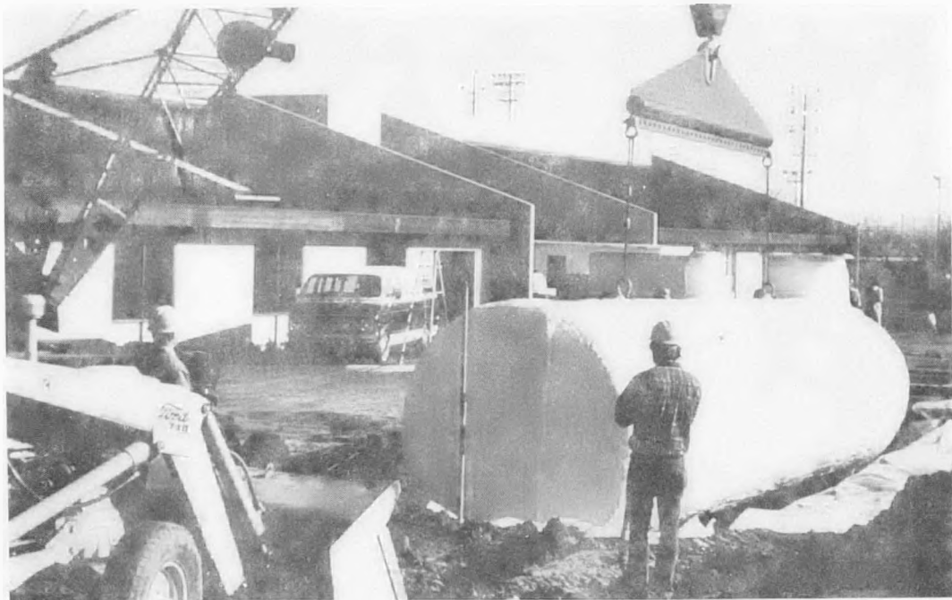
Fig. 3-22 Ground Placement of Tank
