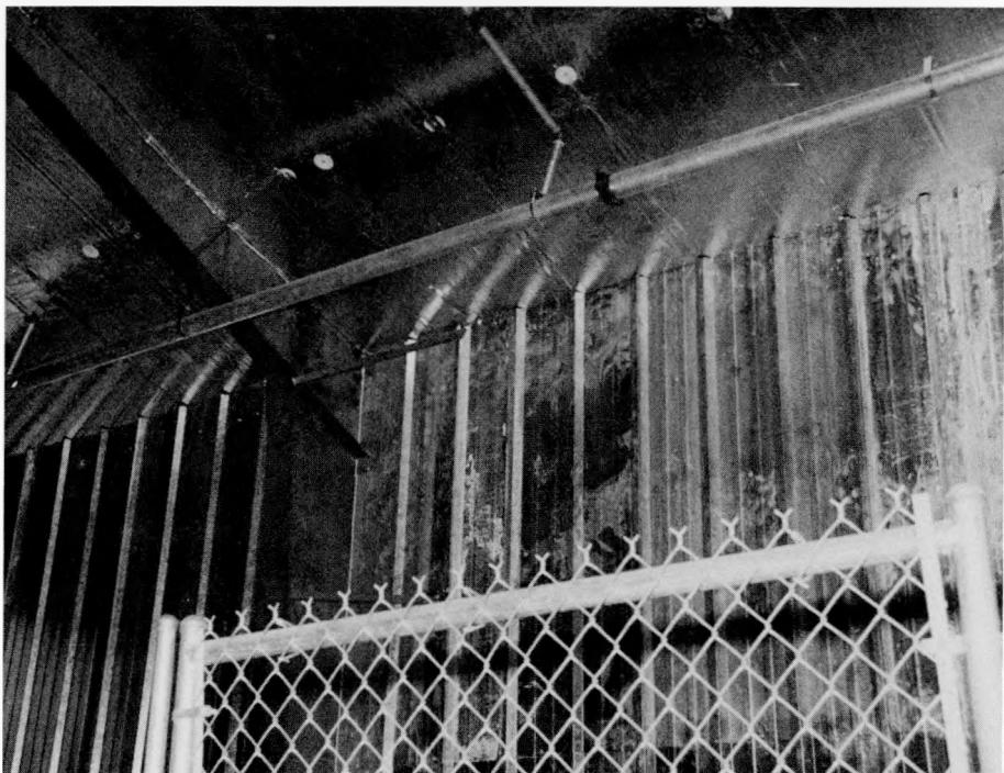
*At the Naval Reactors Facility Site (Idaho Falls, ID), Building 631 was retrofitted with insulation. Fiberglass battings and foil faced foam board were applied to the interior of the roof and walls, with metal ribbed siding protecting the wall insulation, as shown in this picture. The insulation was installed to reduce the heat loss and is estimated to save 2.48 billion British Thermal Units annually.*
