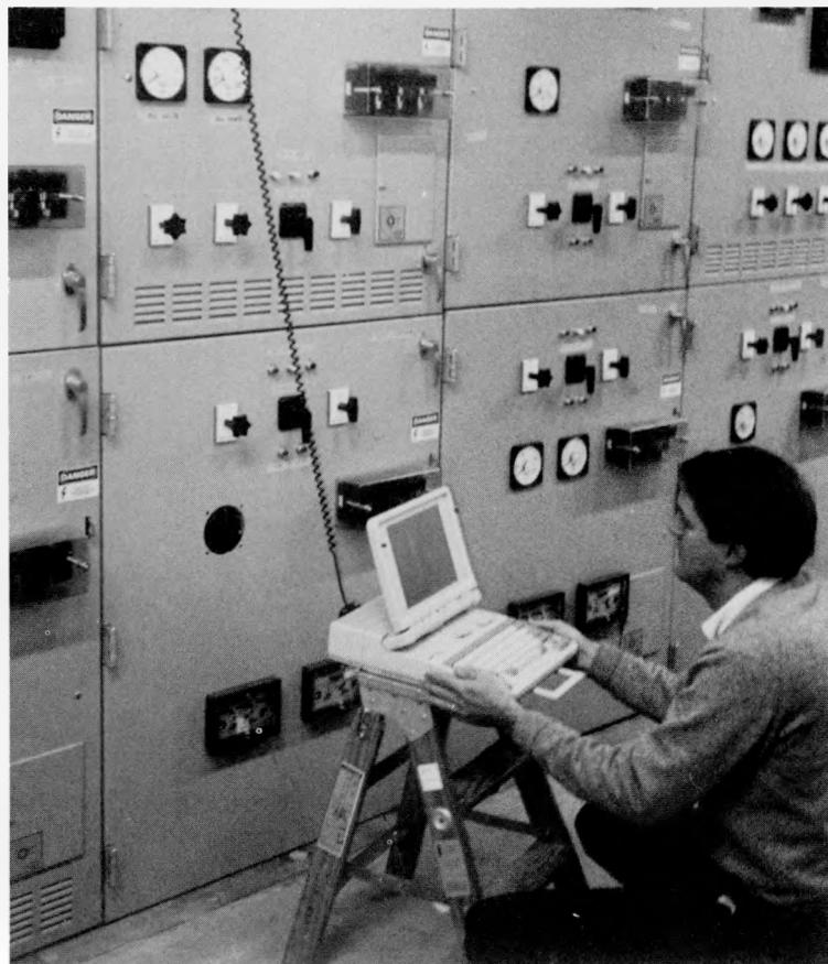
*Pictured is an energy management employee utilizing a Programmable Power Meter Installation at the Lawrence Livermore National Laboratory Main Substation — B-424. This multifunction meter provides instantaneous readouts and historical storage of all electrical variables to pinpoint energy costs and conservation opportunities.*
