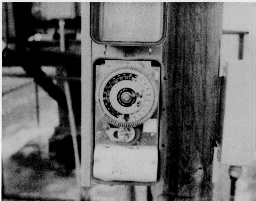
*Pictured is a typical oil well time clock control used at Naval Petroleum Reserves in Colorado, Utah, and Wyoming to reduce electrical demand.*
