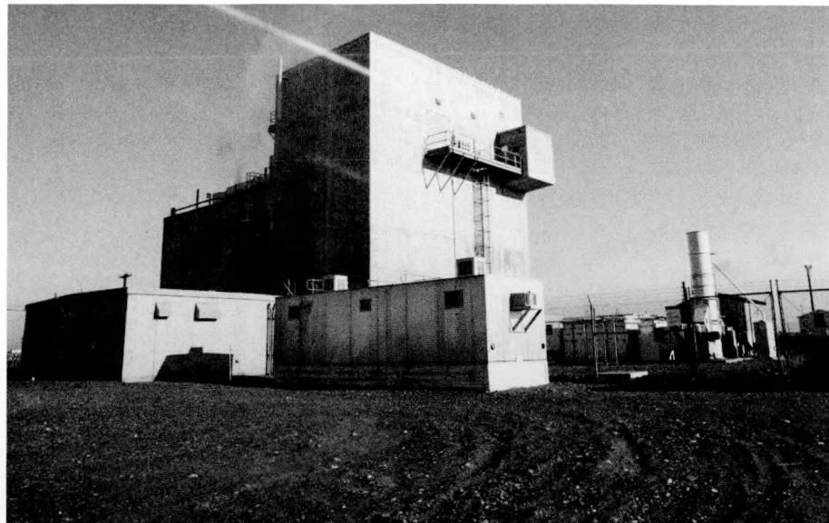
*A study was performed to determine the feasibility of reducing the airflow rates in the 242-S Evaporator Building at the Richland, Hanford Site. This study indicated that a savings of \$27,000 per year could be achieved by reducing lighting in the zones, turning off the domestic water heaters, and turning off the steam to the turbine on the backup exhaust fan.*
