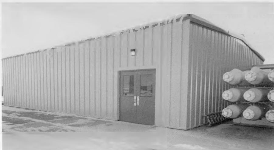
*This Advanced Test Reactor Waste Heat Recovery System at the Idaho National Engineering Laboratory will remove approximately 5000 gallons per minute of secondary coolant from an existing 36" underground pipe, running from the Advanced Test Reactor primary heat exchangers to the cooling tower. The warm secondary coolant (at a temperature between 120°F and 140°F) will be used to provide space heating in 13 of the major buildings at the Test Reactor Area.*
