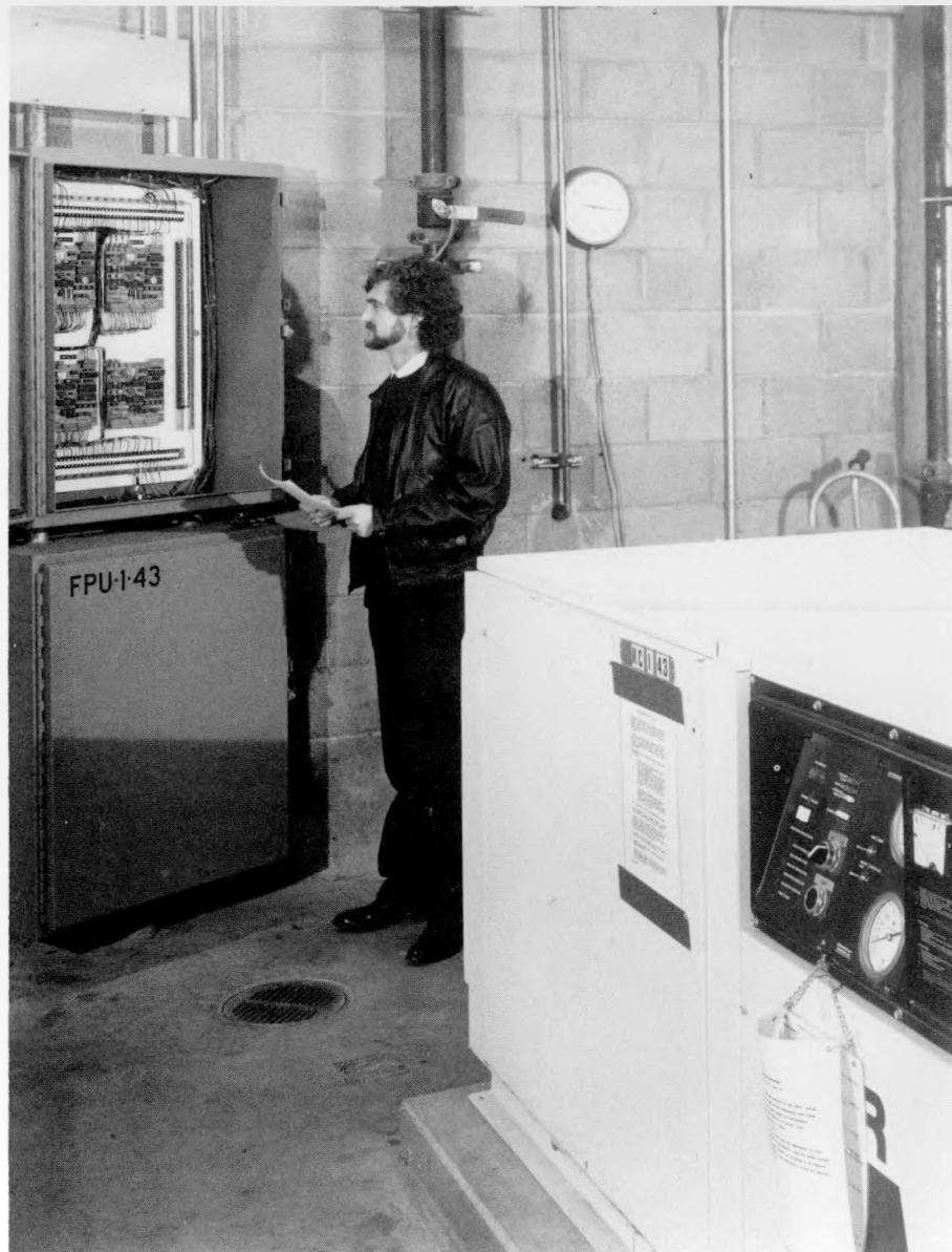
*A Lawrence Berkeley Laboratory, In-House Energy Management staff member monitors flow rates for open lines, and leaky valves at Lawrence Berkeley Laboratory's Compressed Air Facility. The automated control system reduced compressed air consumption by one-third, saving about \$20,000 a year in energy costs.*
