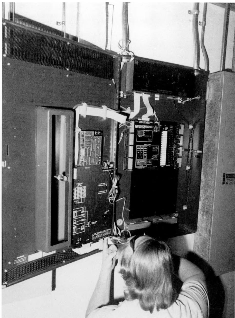
*Pictured is the Andover Controls AC256 Master Plus microcomputer based programmable controller at the North Las Vegas facilities. This energy monitoring system resulted in an estimated annual energy savings of 16,369 million British Thermal Units.*
