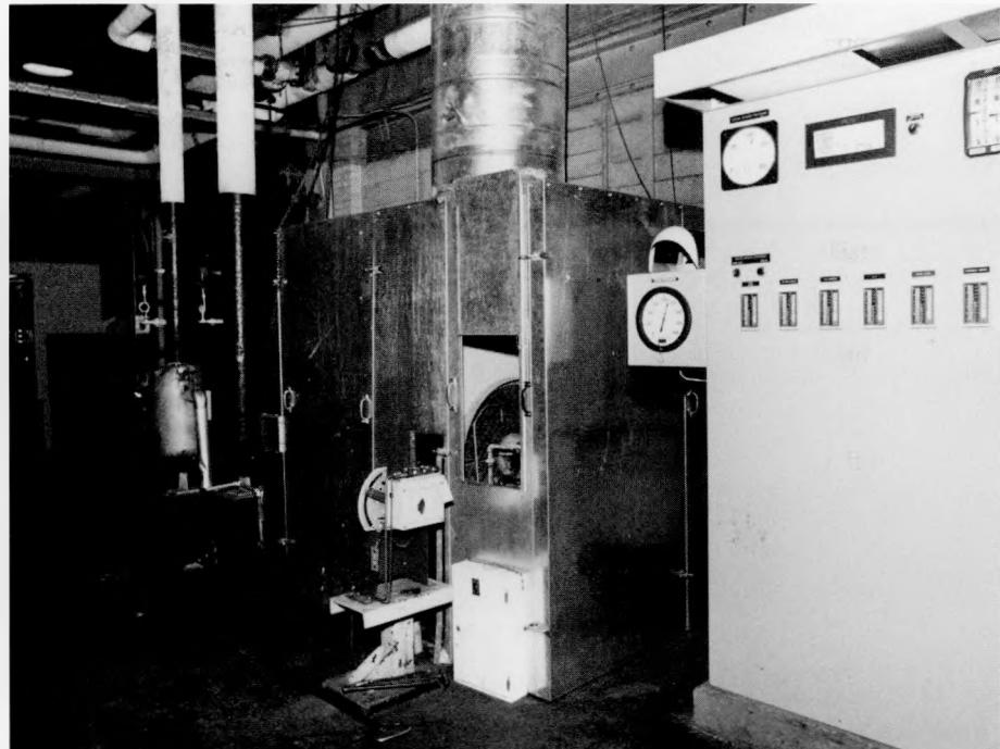
*The Boiler Efficiency Improvement Mockup Plenum was developed at the Hanford Site to determine the final design of the plenum, which would permit full maintenance and maintenance checks to be performed. The 200-E Boiler Efficiency Improvement Project is to provide ductwork to be installed in the steam plant to route hot air from the plant ceiling region to the inlet side of the forced draft fans that supply air into the boilers.*
