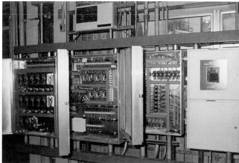
*Shown is the control panel at the Argonne National Laboratory-East's central chilled water plant, containing Direct Digital Controls for optimizing the chilled water plant operation.*
