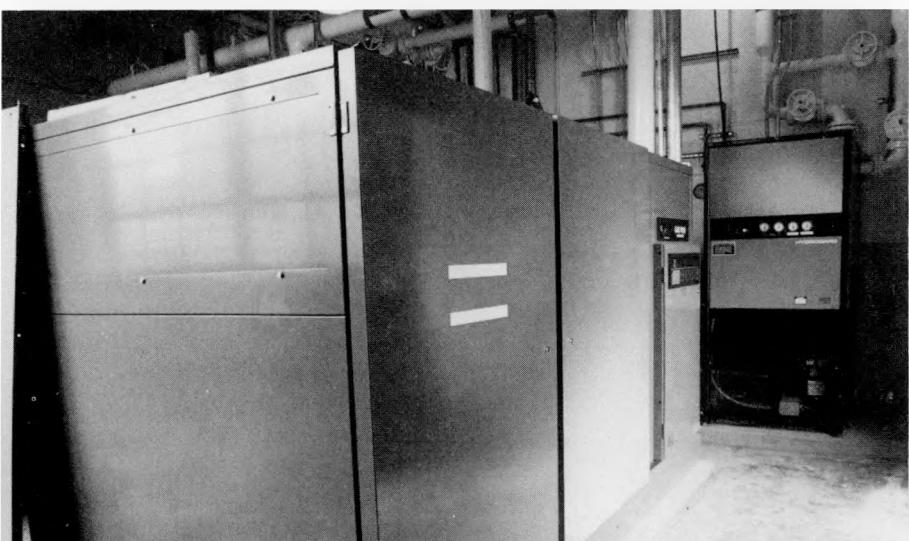
*Shown is one of the two, new central plant air compressors installed at the Bettis Site (West Mifflin, PA). The new, replacement units, provide primary and backup capability and are estimated to save about 500 million British Thermal Units annually as compared with the older, less efficient air compressors.*
