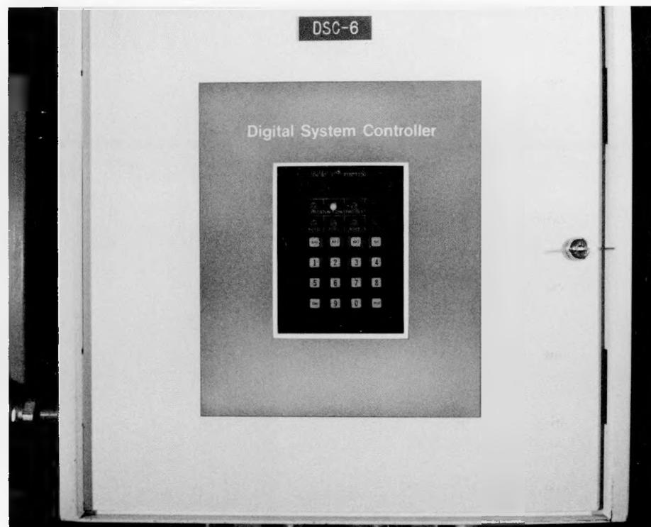
*Shown is a Digital System Controller, for the Heating, Ventilating, and Air-conditioning System on the Administration and Engineering Building, at the Nevada Test Site. This controller will reduce the electrical consumption 388,000 kilowatthours and produce an annual cost savings of \$21,384.*
