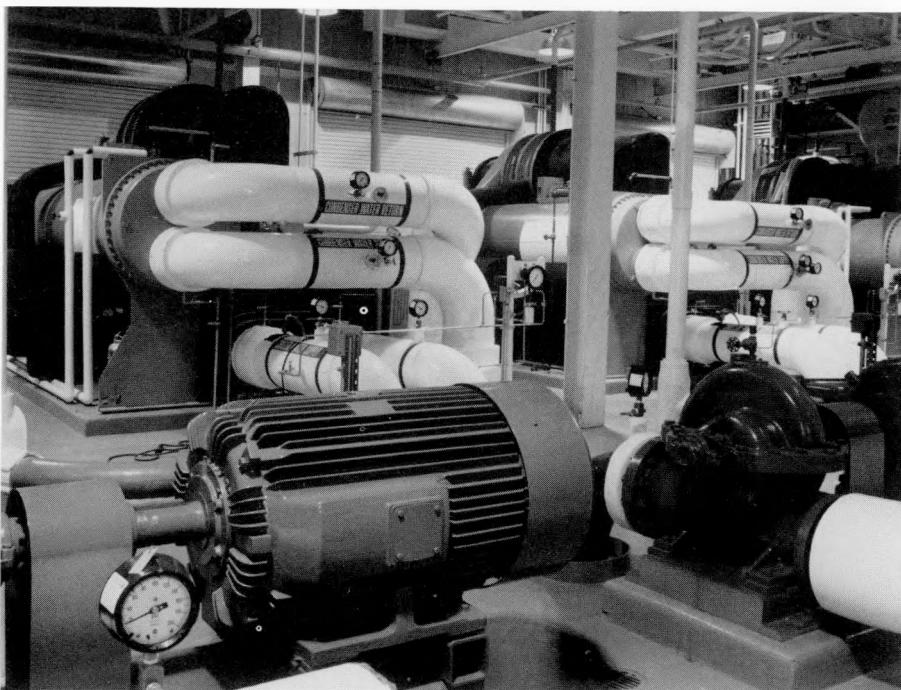
This photo is part of the energy conservation features of the recently completed Central Chilled Water Facility at the Brookhaven National Laboratory, 250 horsepower variable speed chilled water pumps (foreground) and high efficiency 1,250 ton electric centrifugal chillers (background).
