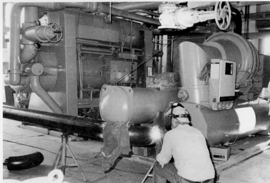
*Pictured is the New Chiller and Free Cooling Heat Exchanger being installed at the power plant of the National Institute for Petroleum and Energy Research Center. This new system will save approximately \$1,500 per year in energy costs.*
