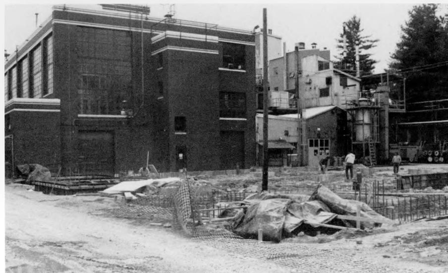
*Shown is Building 84 renovation at the Pittsburgh Energy Technology Center, featuring inefficient glazing to be replaced by energy conserving brick and insulated block system.*
