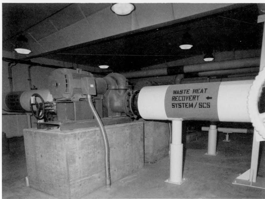
*Either of two main distribution pumps as shown here will be used to circulate the secondary coolant water through the Advanced Test Reactor Waste Heat Recovery System loop. A small third pump will be used to circulate 200 gallons per minute of coolant through the loop to prevent freeze up in winter when the Advanced Test Reactor is not operating.*
