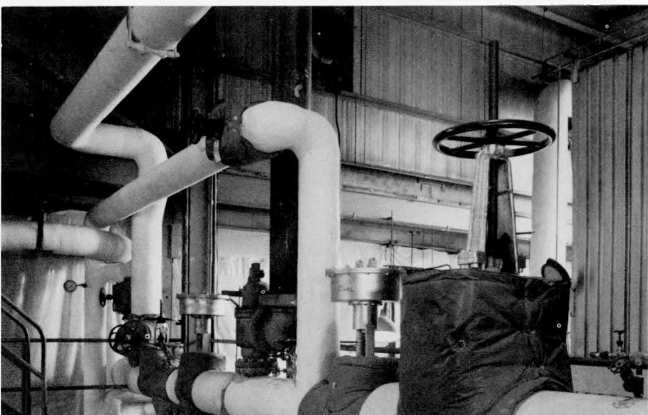
*This photo is representative of insulation upgrades completed on piping in numerous buildings throughout the Brookhaven National Laboratory Site.*
