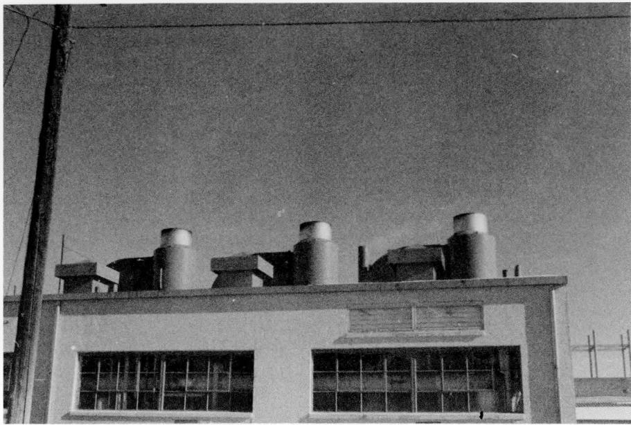
*Shown is the Central Heating Plant Boiler House at the Naval Reactors Facility Site (Idaho Falls, ID). The three chimneys and main combustion chambers of the Naval Reactors Facility boilers were sand blasted to clean the combustion products off the heat transfer elements. This sand blasting is estimated to save 3.54 billion British Thermal Units per year.*
