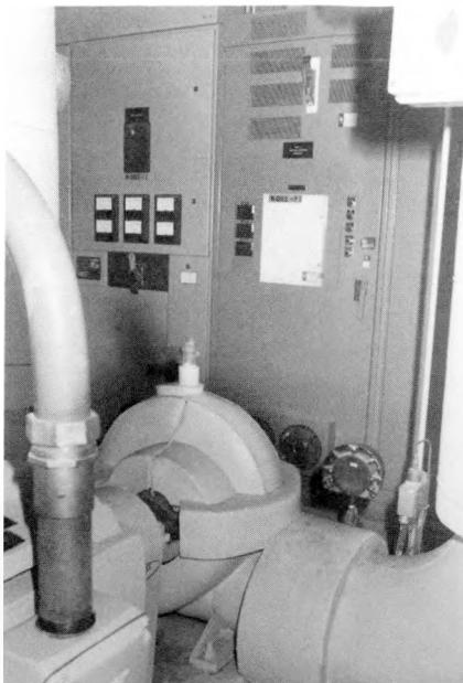
*Pictured is the variable frequency drive and one of the chilled water distribution pumps at the Argonne National Laboratory-East's central chilled water plant. The drive saves pumping energy as chilled water flow to the buildings is reduced with a reduction in the building cooling loads.*
