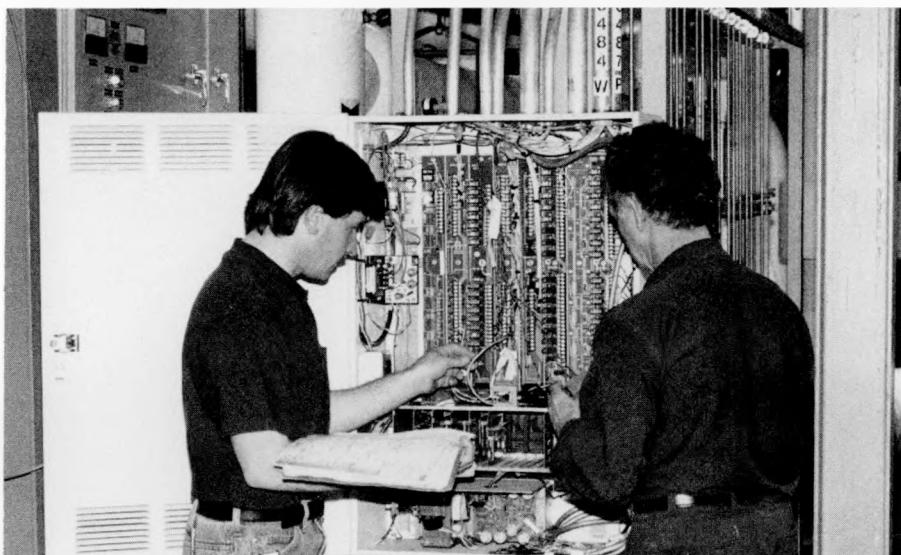
*Electrical Technicians at Princeton Plasma Physics Laboratory are completing wiring to the in-field Remote Computer Unit which receives its commands from the main Computer Unit, the Energy Management Control System.*
