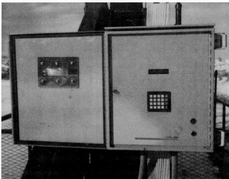
*Pictured is a typical oil well automatic pump-off controller used at Naval Petroleum Reserves in Colorado, Utah, and Wyoming and Naval Petroleum Reserves in California for the optimization of oil well artificial lift units.*
