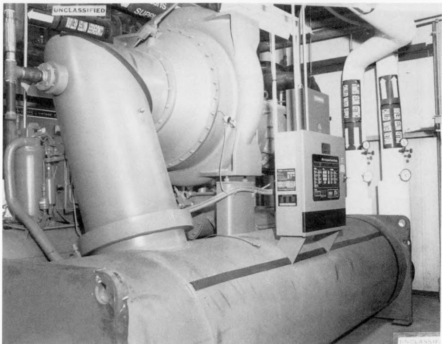
*Pictured is the new 450 ton "York" chiller unit installed in FY 1989 at Knolls Atomic Power Laboratory. This unit replaces older, less efficient reciprocating chillers which serve the Knolls Atomic Power Laboratory computer complex.*
