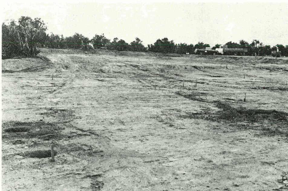
Fig. 2. Rough grading of array field.
