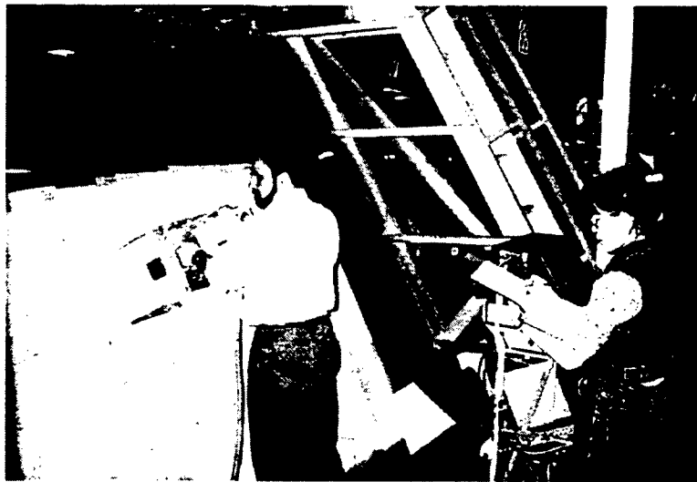
(b) Application of Thermography on 747 Aircraft
