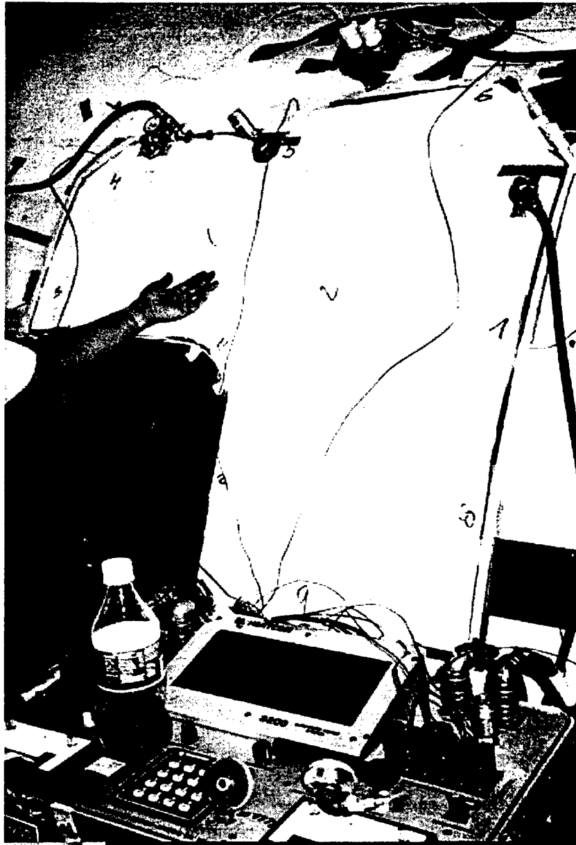
Figure 8: Doubler Cure Process - Heat Blanket, Insulation, and Vacuum Bag Assembly
