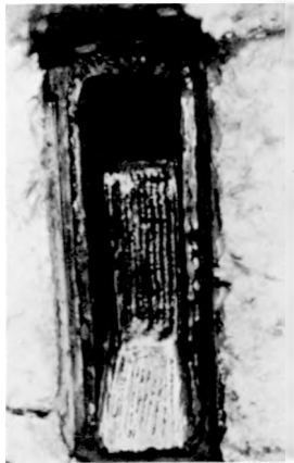
(c) PARTIAL GRINDING STARTED ON FIRST LAYER ("BUTTER")
