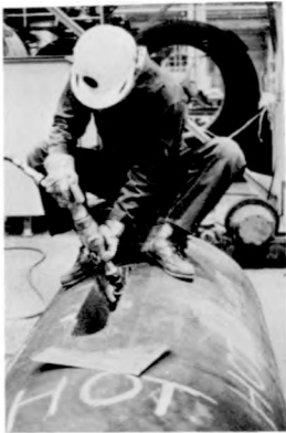
(c) GRINDING TO REMOVE FLAME EFFECTS
