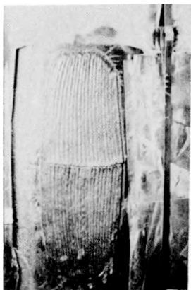
(e) FINAL WELD CROWN PASS COMPLETED
