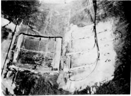
BACKING STRIP AND INTERIOR GAGES IN PLACE
