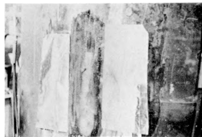
(f) FINAL WELD CROWN PASS AFTER GRINDING; GAGE AND THERMOCOUPLE COVERS IN PLACE
