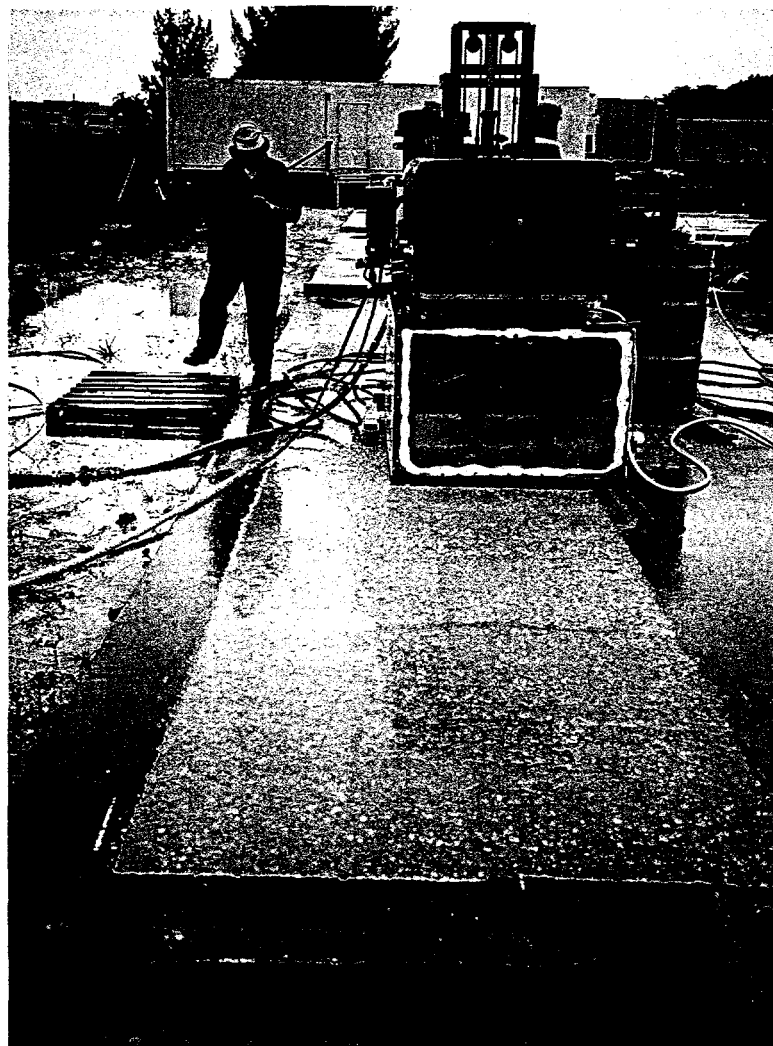
Figure 7.8 Lot B scabbling; wet, after-rain concrete surface a) At the beginning of the second row b) In the middle of the second
