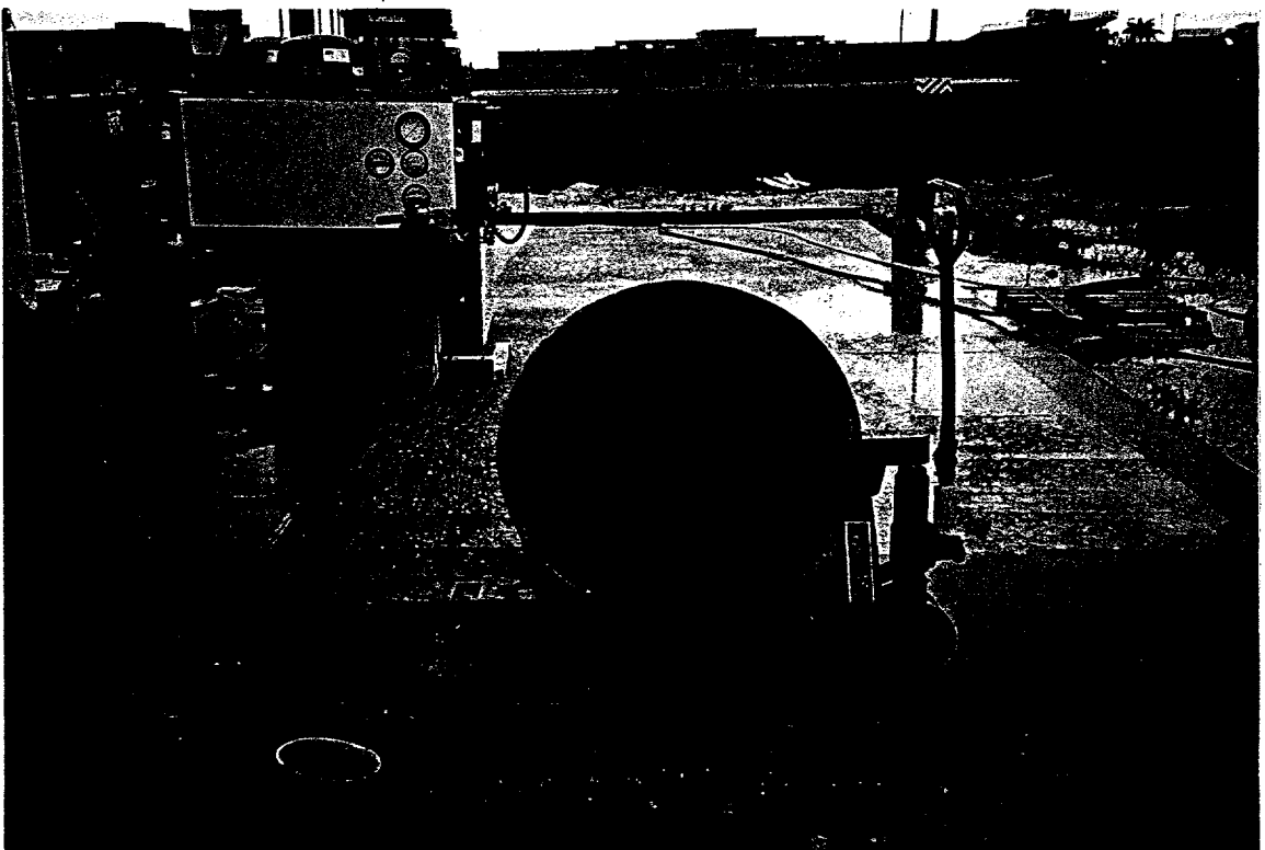
Figure 7.14 Wet concrete debris collected in the drum is discarded when it is ~1/2 full (or whenever it is convenient, e.g. at the shift or the raw end)
