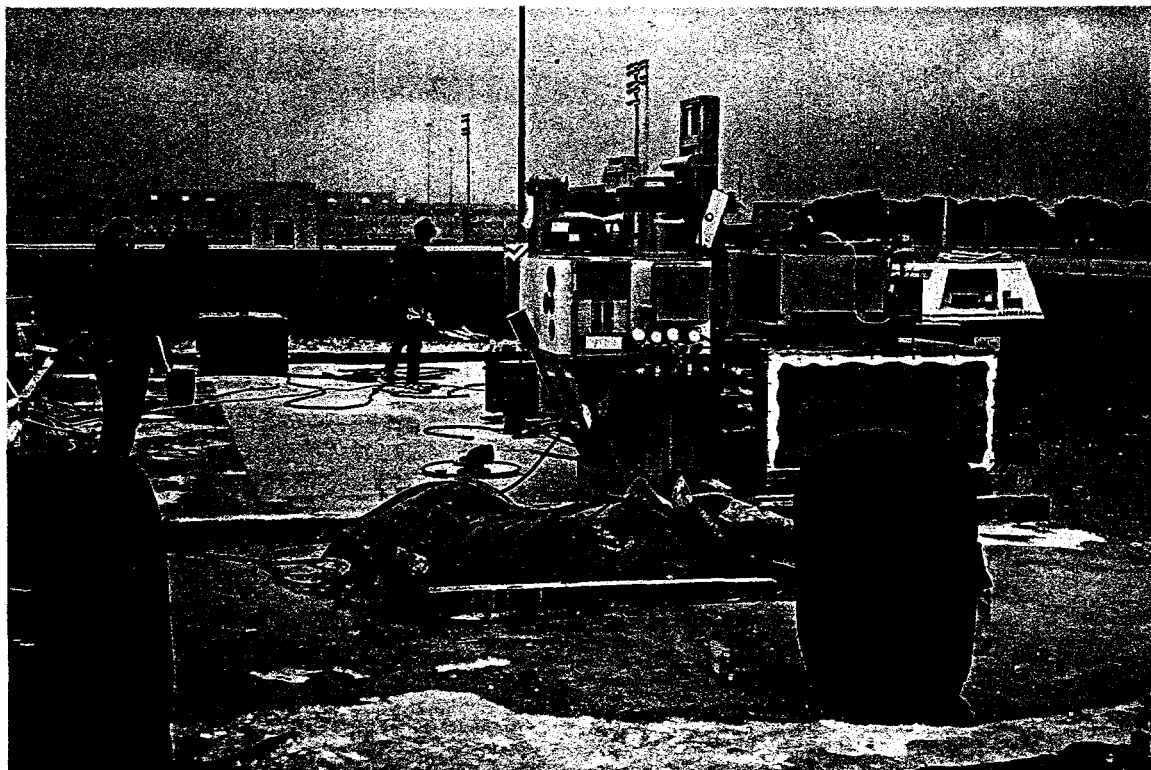
Figure 7.10 Lot B scabbling is finished, equipment diss-assembly/packing starts Acc mulated concrete debris is stored under blue tarpoline in a forefront
