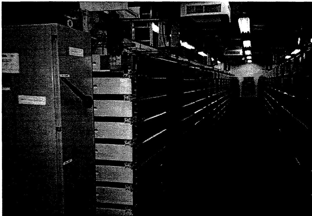
Figure 2-15. Completed Vernon Facility Battery Room.
