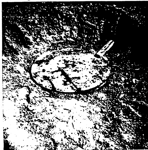
VIEW OF COVERED CORRUGATED PIPE WITH \frac{1}{2} " STEEL COVER.
