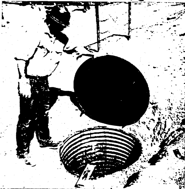
VIEW OF CORRUGATED PIPE WITH THE \frac{1}{2} " STEEL LID OPEN
