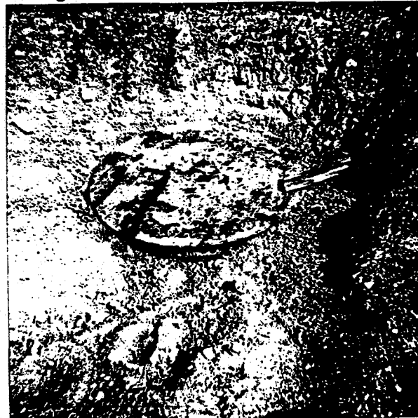
VIEW OF \frac{1}{2} " STEEL LID COVERING CORRUGATE PIPE SET IN GROUND FOR WASTE OIL DISPOSAL.
