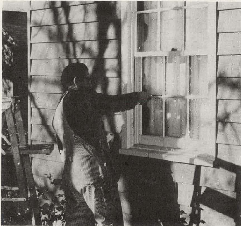
Figure 5. Storm Window Installation
