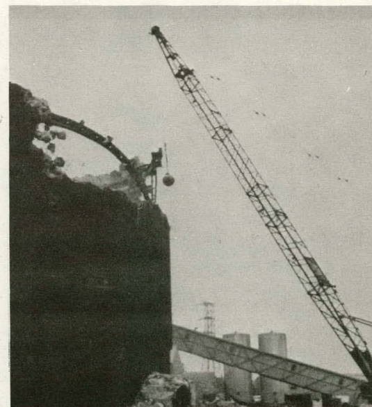
BALLING OPERATION - POLAR CRANE RAIL
