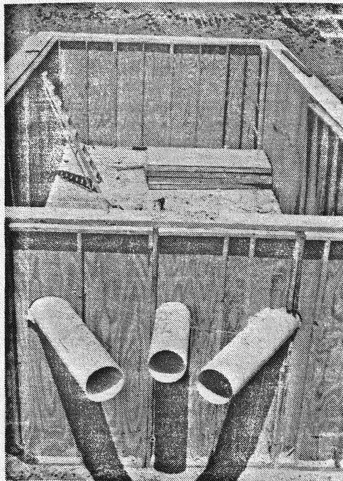
Figure 18: Placement of Digester Discharge Pipes
