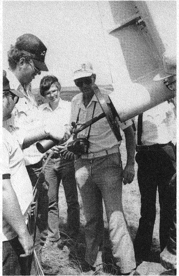
Figure 12. Preparation of Nacelle Section Prior to Assembly.
