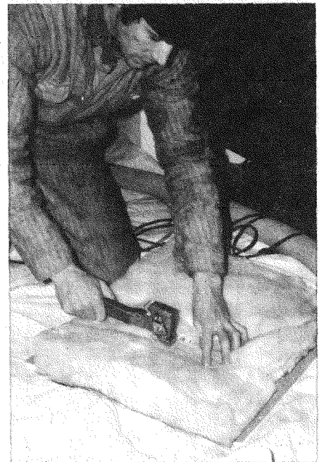
INSULATION BATT BEING STAPLED ONTO ATTIC FLOOR TRAP DOOR, PART OF PRINCETON RETROFIT PACKAGE A.
