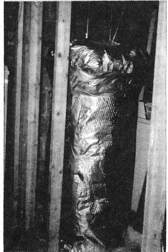
ELECTRIC HOT WATER HEATER FOLLOWING RETROFIT. WRAPPED IN FOIL BACKED R-7 INSULATION.
