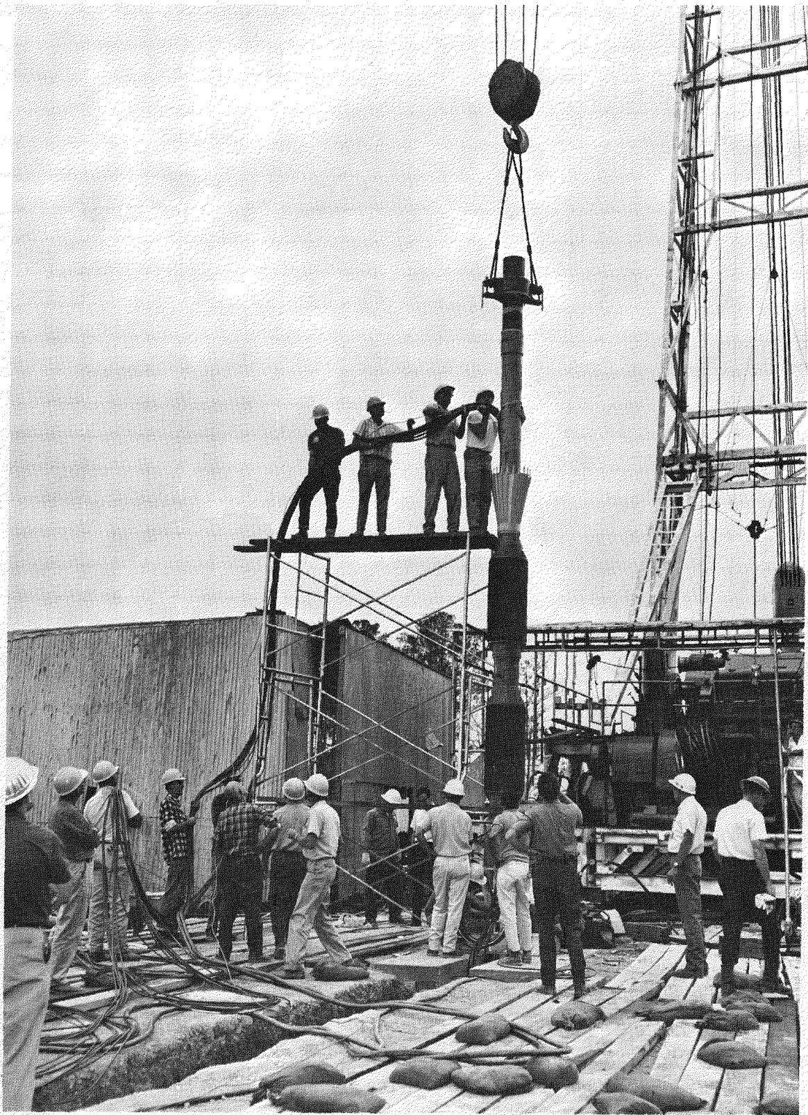
Figure 2-13 Lowering the Packer Assembly
