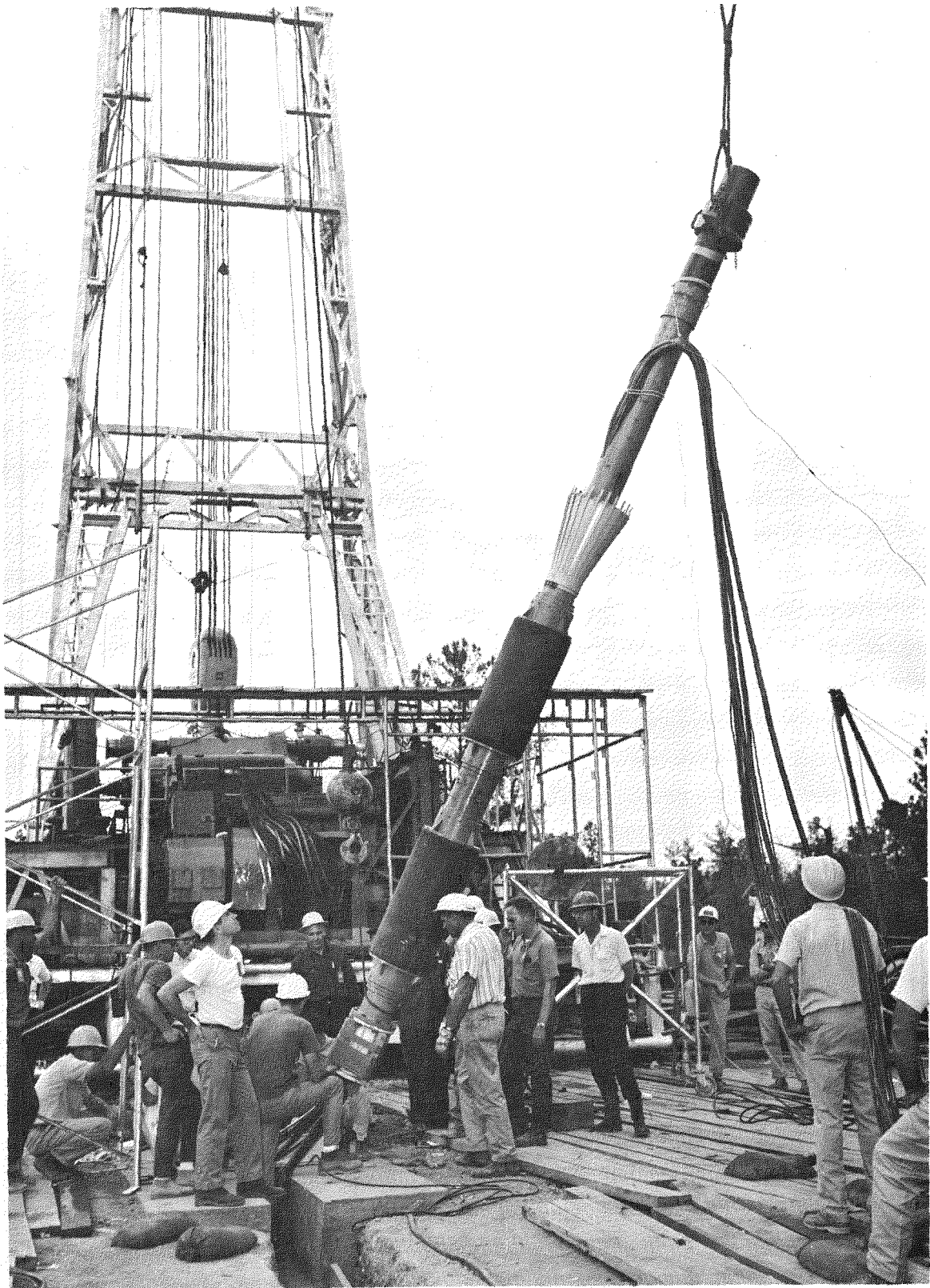
Figure 2-12 Preparing to Lower the Packer Assembly
