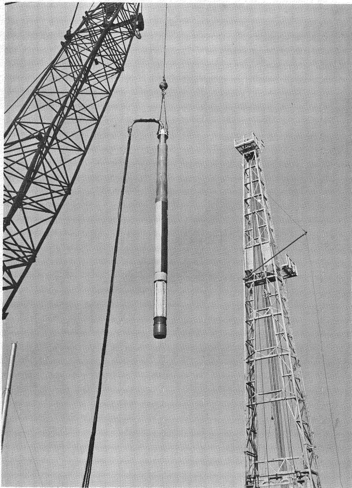
Figure 2-9 Device Package Being Lowered into the Emplacement Hole
