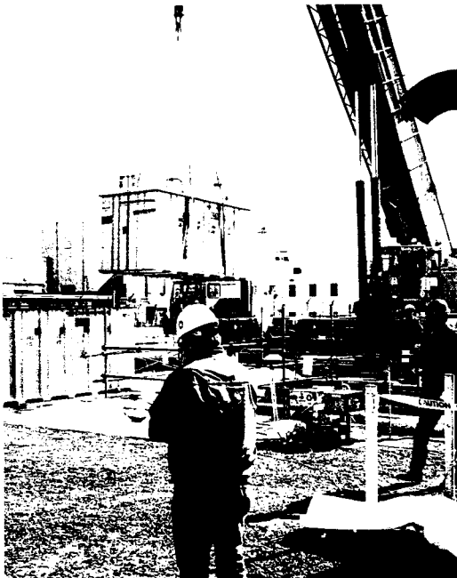
Figure A-9 Three of four IX columns positioned in waste container. (96050241-15)
