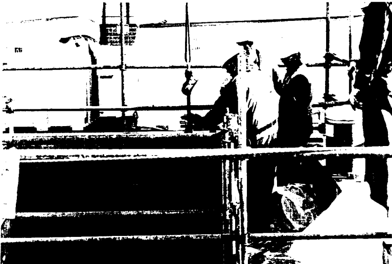
Figure A-6 Absorbent added to empty IX columns. (96050172-11CN)
