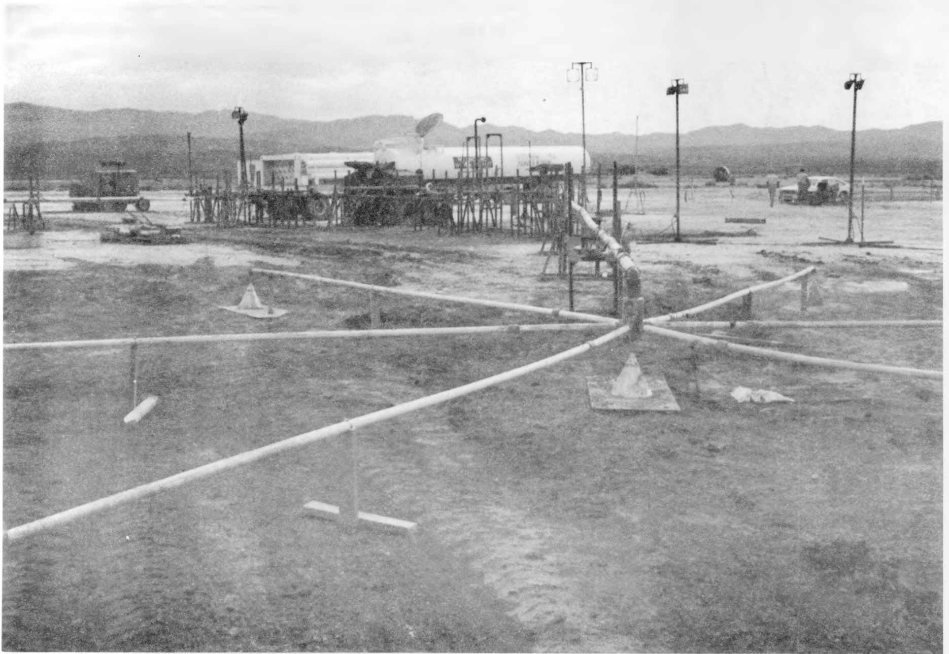
FIG. 4. The N_2O_4 Spill Facility with the Multi-exit Spill Configuration.
