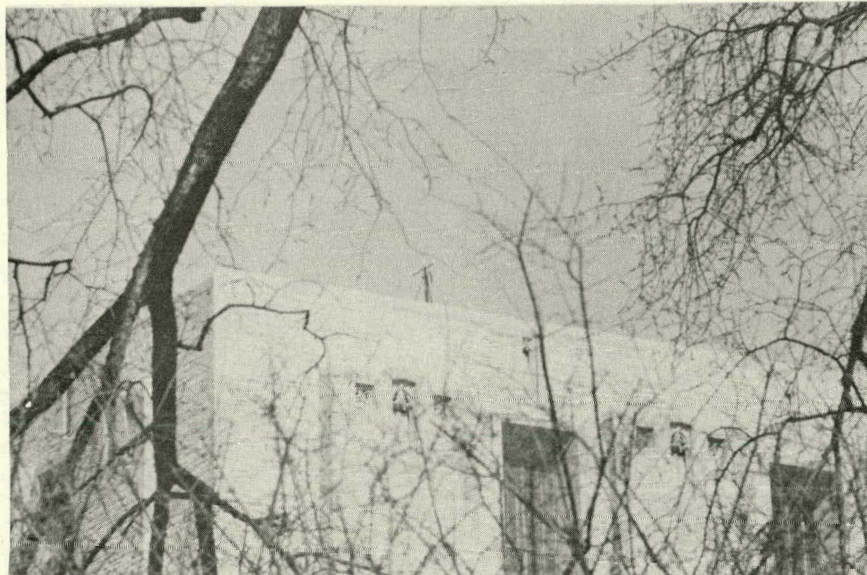
FIGURE H.2 View Looking Northeast toward Anemometer on Roof from Ground
