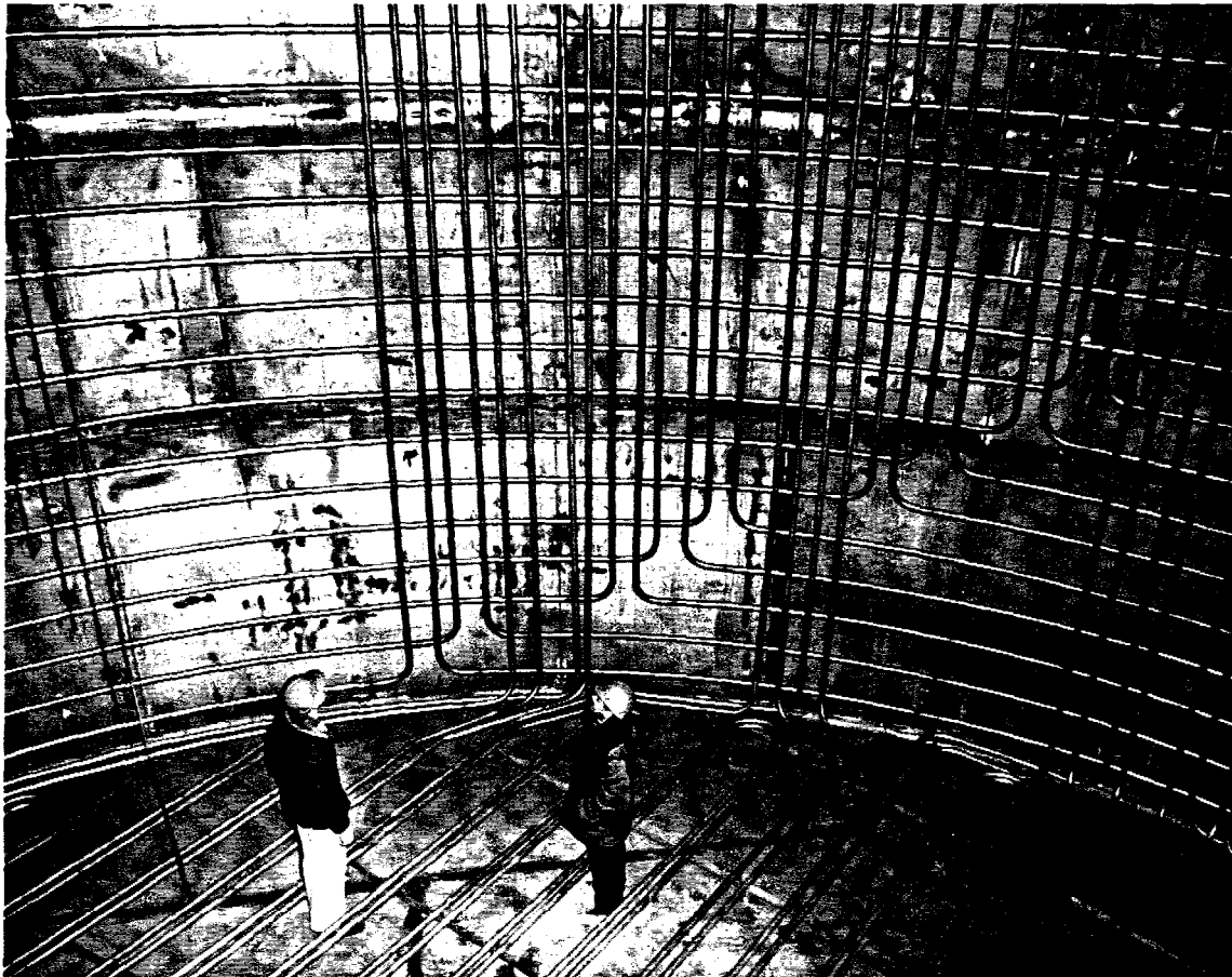
Figure 14. Cooling Coils Lining the Walls and Floor of the High Level Liquid Waste Tanks at INEEL.
