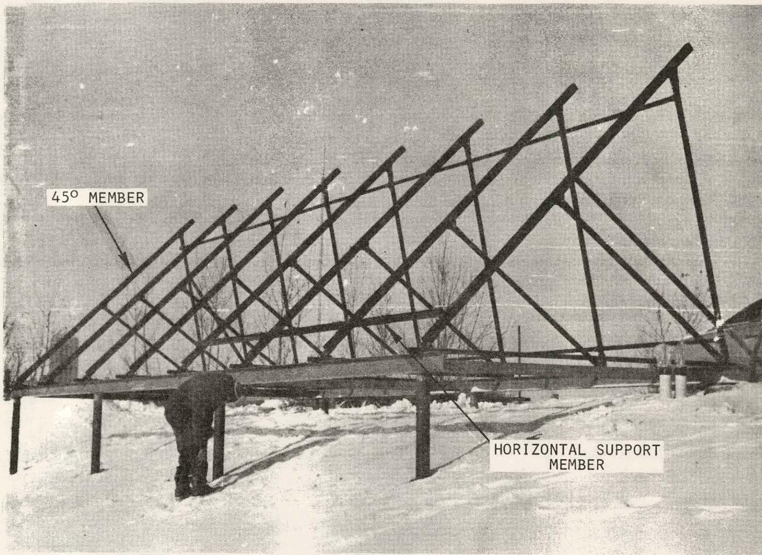
Figure 2. Harding A-Frame Structure Showing Horizontal Support Member
