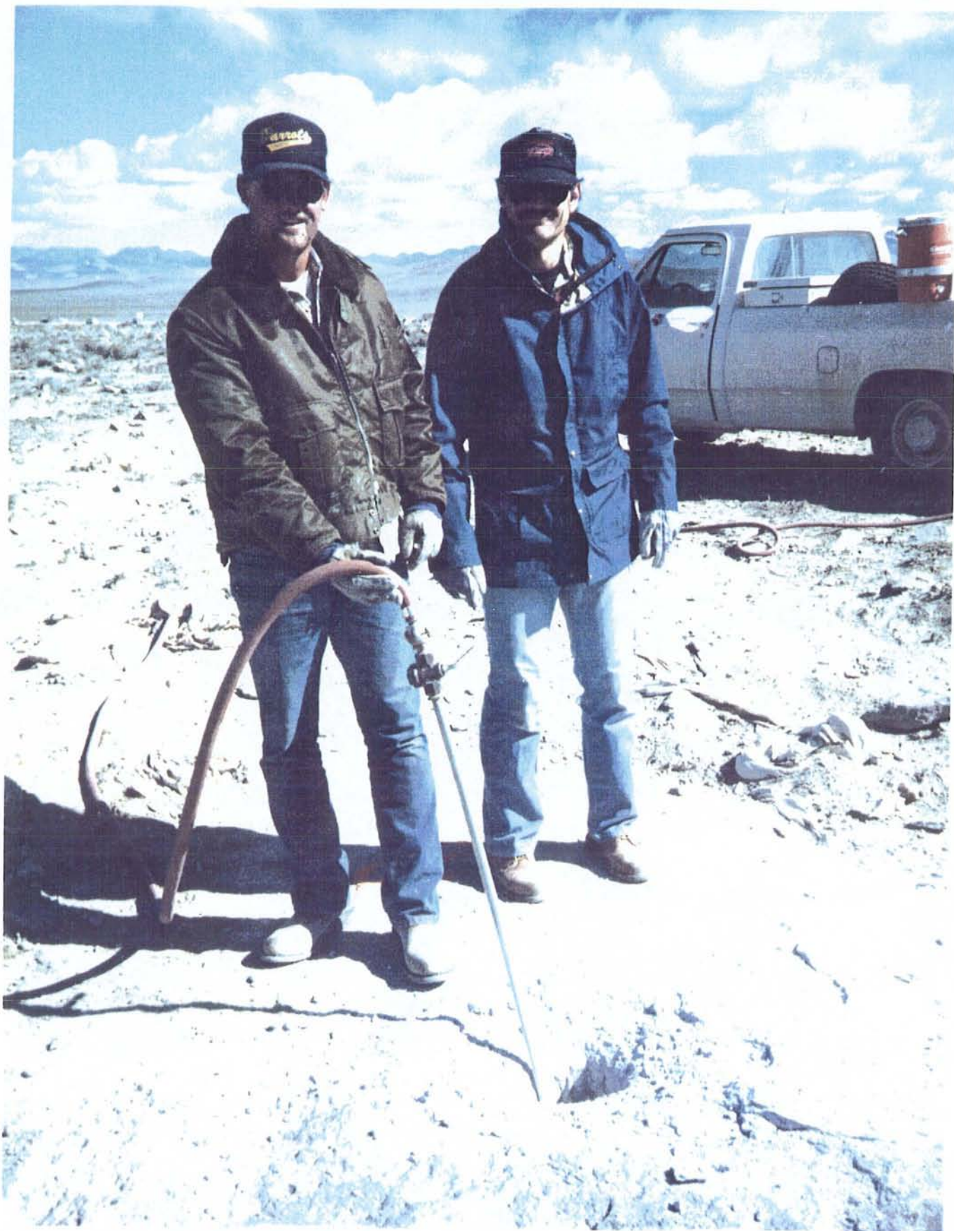
Figure 6. Steel, Hollow Tube With High Pressure Hose Attached For Cleaning Holes in Tuff Formation
