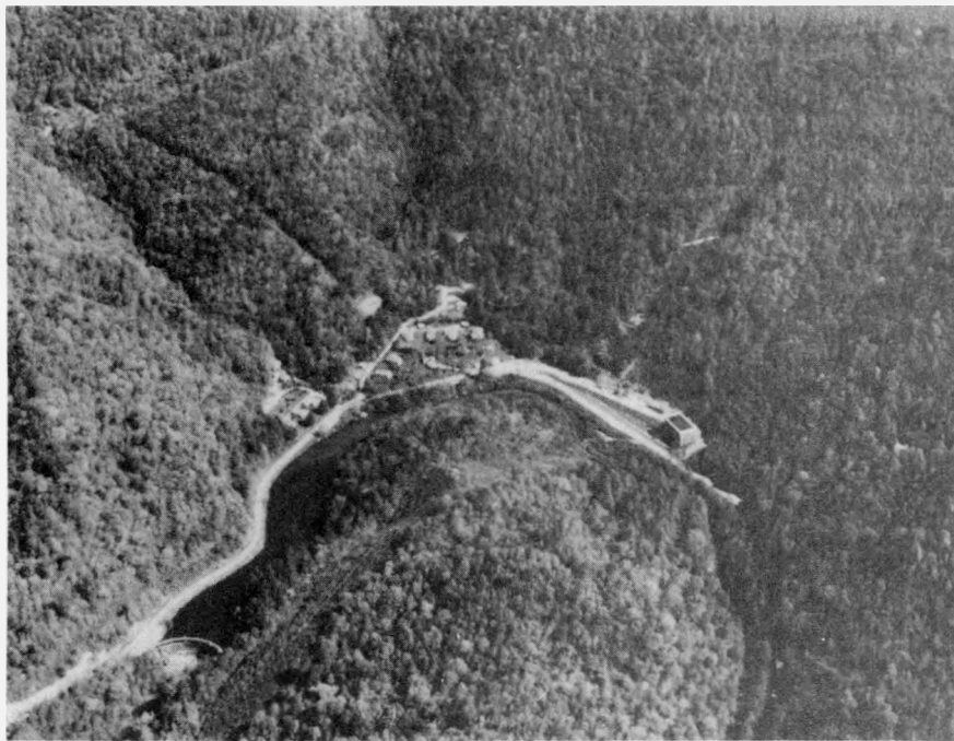
Figure 12. Thorpe powerhouse, and Tuckaseegee dam and reservoir
