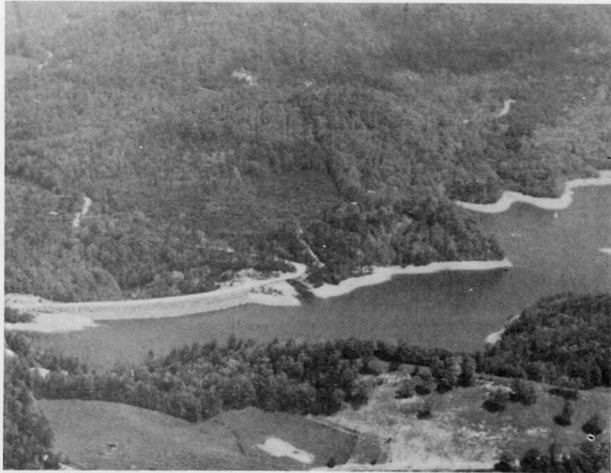
Figure 8. Wolf Creek dam and reservoir, viewed from upstream
