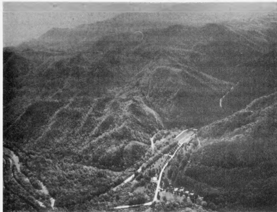
Figure 16. View of Nantahala powerhouse
