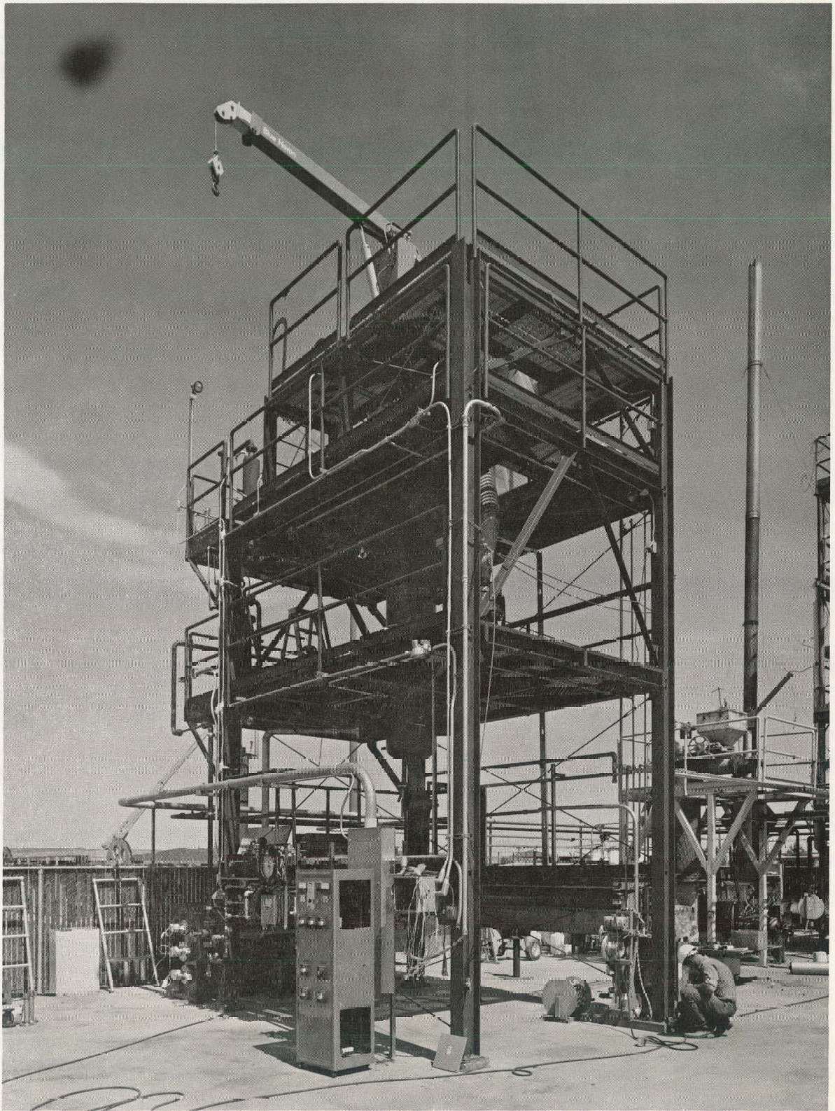
FIGURE 15. PDU Without Gas Preheater
