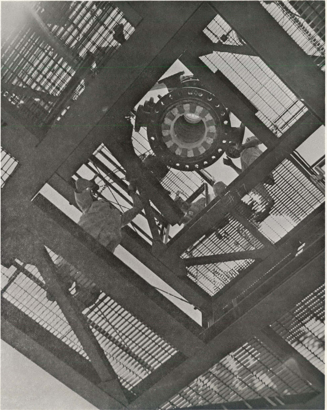
FIGURE 14. View of Main Section Showing Lining and Insulation
