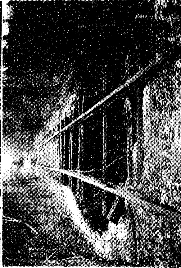
B) WASHOUT AREA 34' Length x 12' Depth North of ABANDONED water PLANT.
