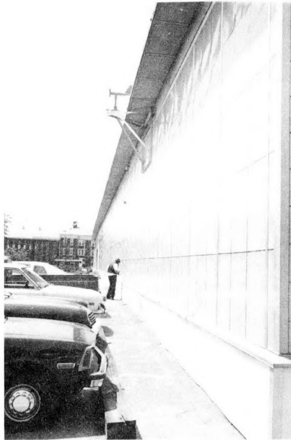
Figure IV-B-1 Passive Solar Wall
