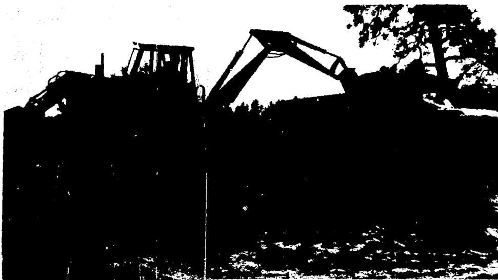
Fig. 6.10. Excavation with backhoe. Soil is loaded directly into a dump truck.
