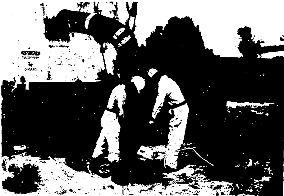
Fig. 10.3 Collection of contaminated soil with vacuum cleaner.
