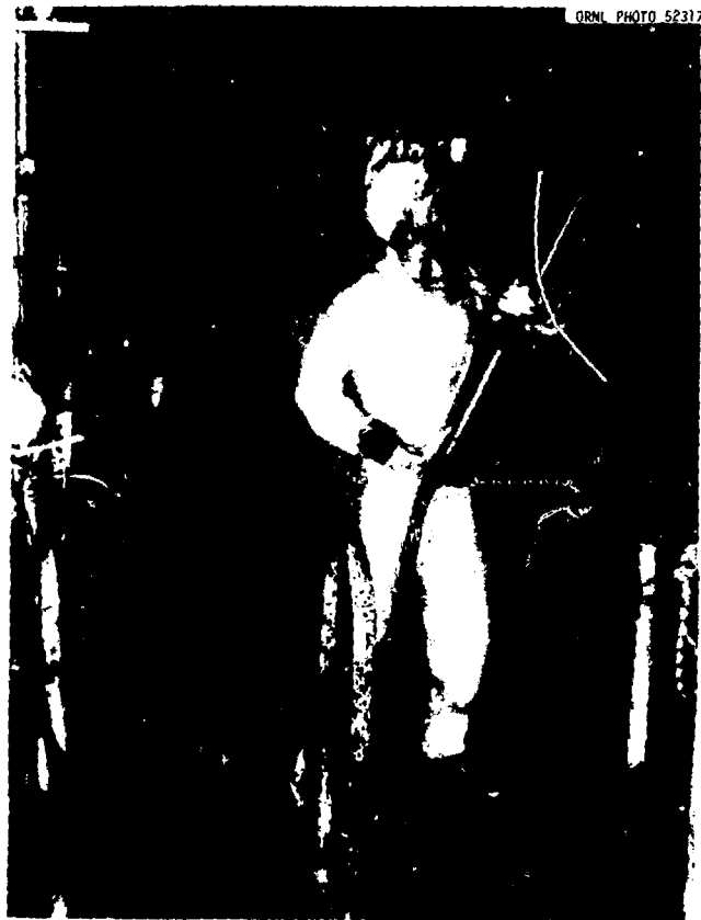
Fig. 15.9. Steam jet flushing of 3019 cell.
