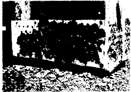
Fig. 21.11. Spalling done around rebar.
