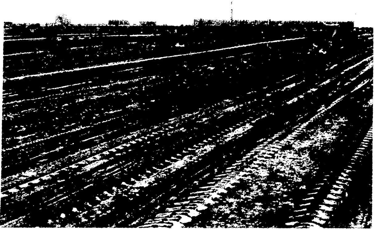
Fig. 17.14. Gravel strips between trenches in second burial ground.
