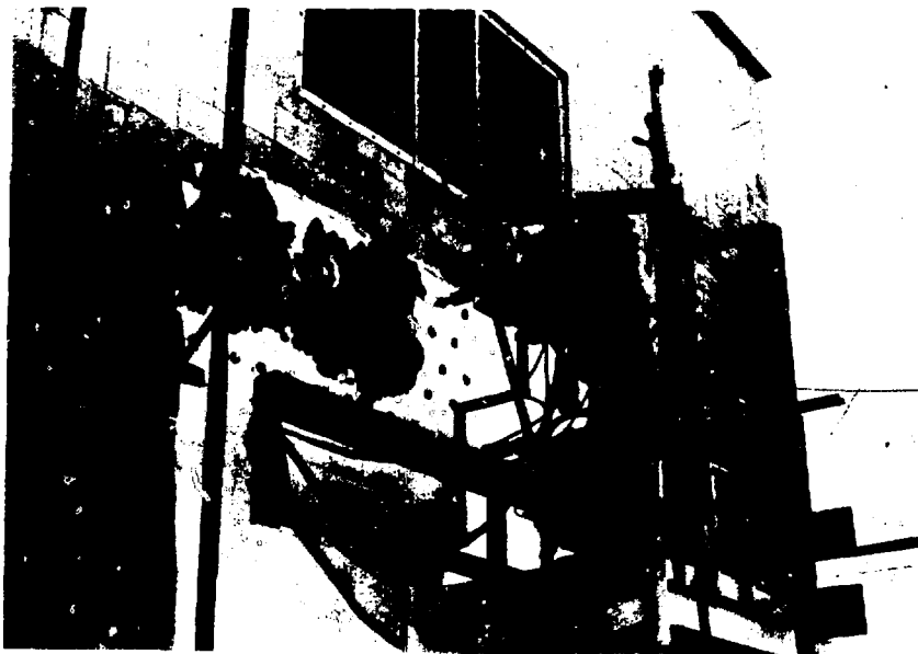
Fig. 21.13. Concrete spaller in operation.
