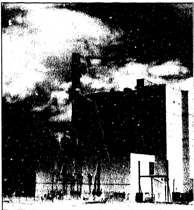
High-sulfur waste coal will be combusted in fluidized bed boilers at the 41.5-MW Colstrip Energy Project. Approximately 261 million kWh of annual energy production from the $97.1 million plant will be sold to the Montana Power Company.
