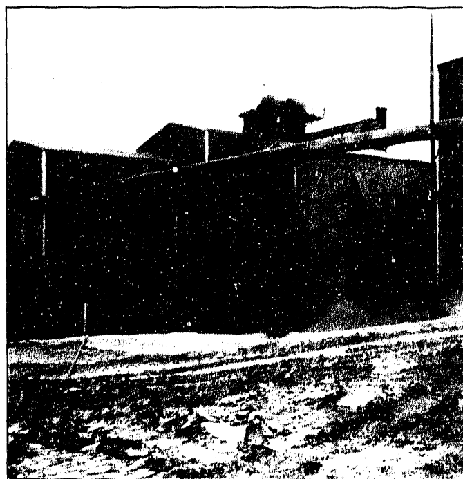
Fuel for the $5.1 million plant is obtained from the adjacent Pacific Crown Timber Products sawmill. Electricity produced is sold to Washington Water Power while extracted steam is used in the sawmill's dry kilns.
