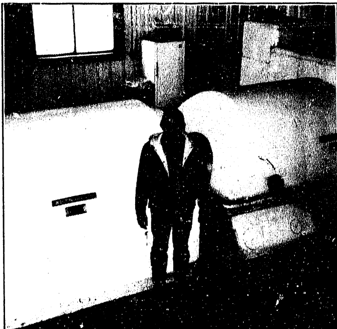
Wood Power, Inc. plant supervisor Rick Bowen stands in front of the steam turbine (right) and 6.2 MW electric generator (left).
