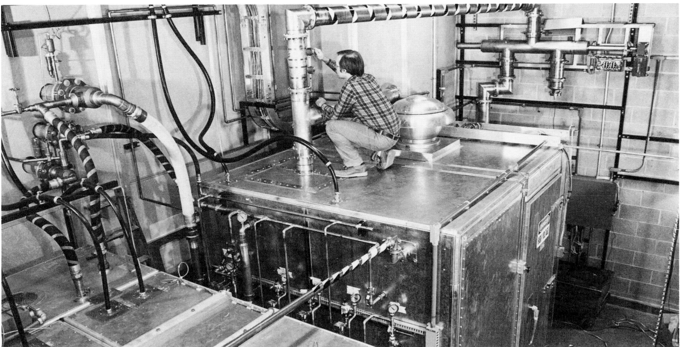
Figure 57. PLT high power ICRF equipment under construction.
