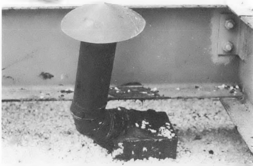
Figure C.21 Vent Pipe Modified to Allow for Solar Collector Installation
