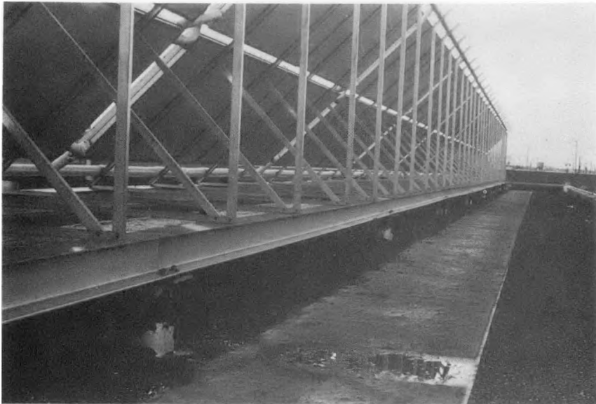
Figure C.31 Coated Felt Walkway on Roofing
