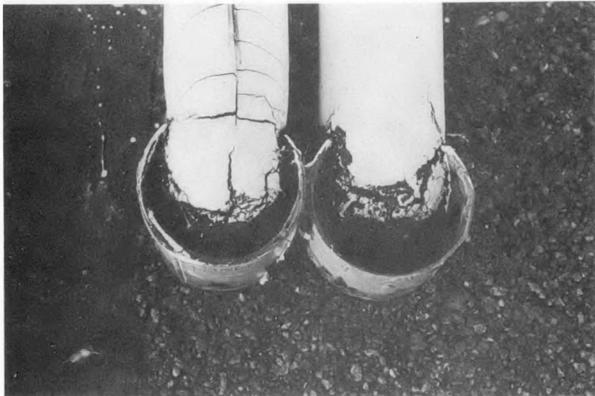
Figure C.16 Pitch Pockets for Pipe Penetrations
