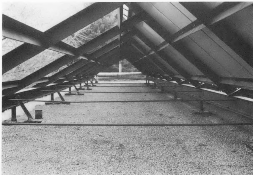
Figure C.4 Steel Columns Extending Through Roofing Support Collector Frames
