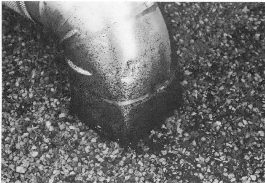
Figure C.14 Pipe Penetration for Which The Type of Flashing was Not Determined
