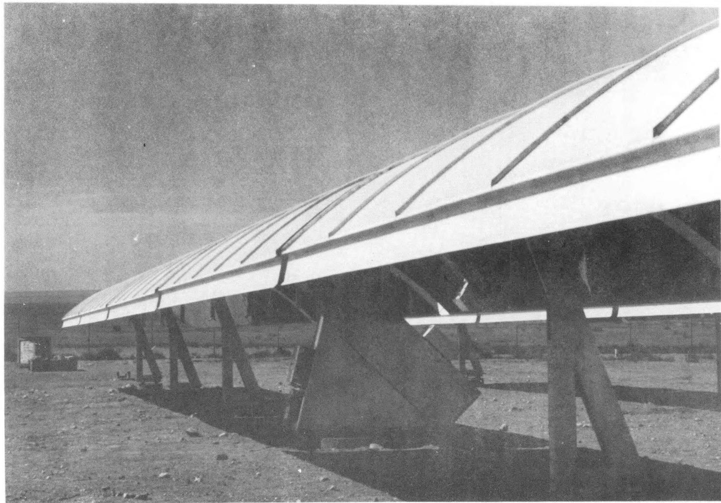
Figure 5 SKI T-800 Parabolic Trough Solar Collector
