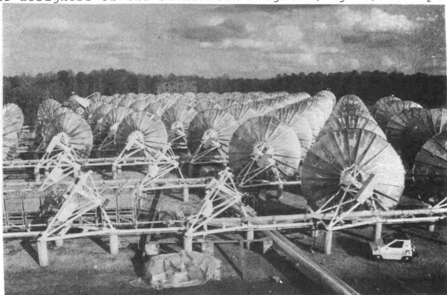
Figure 3 - Construction scene at Shenandoah showing center-field manifold and branch piping.
