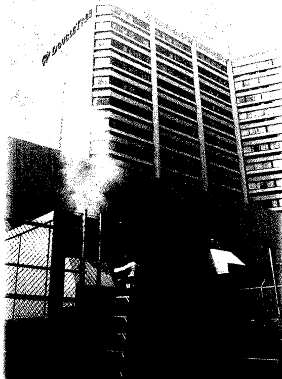
High efficiency and modular construction make fuel cells the power generation system of choice in distributed generation scenarios. The first commercial fuel cell installation in the northwestern U.S., this 200-kW ONSI phosphoric acid fuel cell unit helps to power a Spokane, Washington, hotel.
