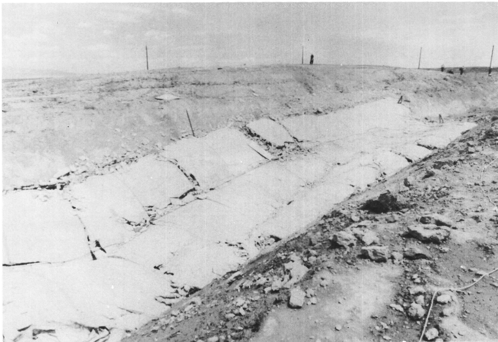
Figure 8. Demolished exhaust stack collapsed in trench.
