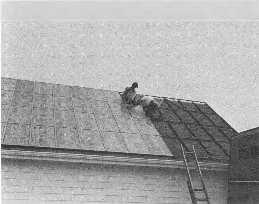
Fig. 16. Solarex PV modules being mounted on the Solarex prototype.
