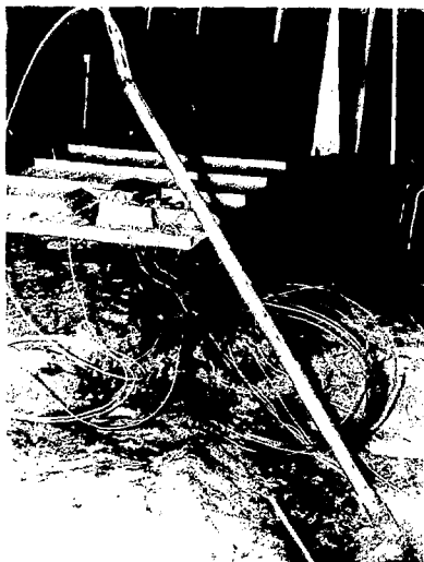
Fig 4.7 Installation of a peripheral heater.
