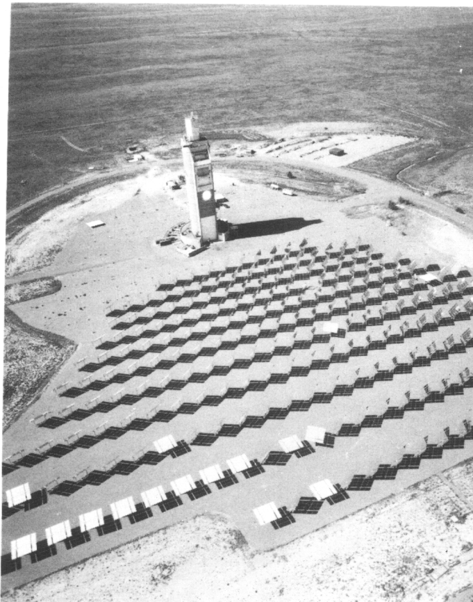
FIGURE 3 AERIAL PHOTOGRAPH OF THE CRTF (with the cavity receiver on the tower)
